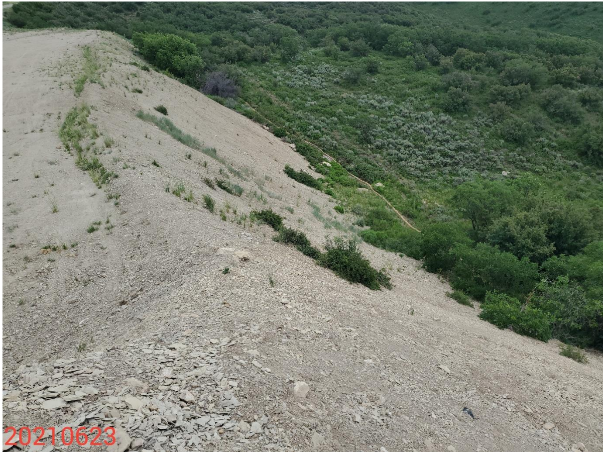
Photo 15: Photo taken from the east end of the Location, facing northeast. Photo shows BMPs to protect and stabilize the slopes of the Location remain missing or insufficient/inadequate.
