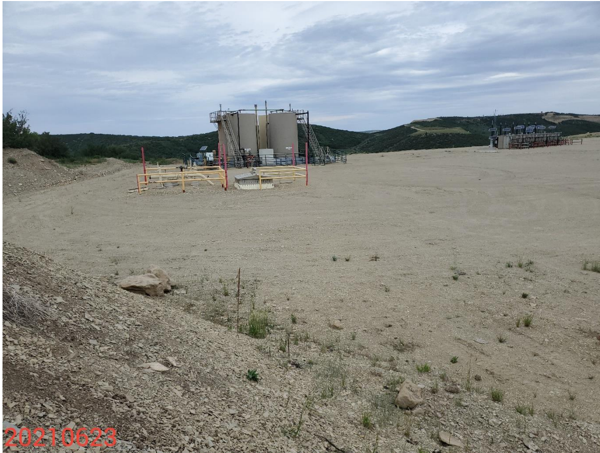
Photo 6: Photo taken from the southwest end of the Location, facing west. Photos 6-8 provide an overview of the Location from west, northwest to north. Photos show interim reclamation of areas not needed for production has not been performed in accordance with 1003 Rules and Corrective actions.
