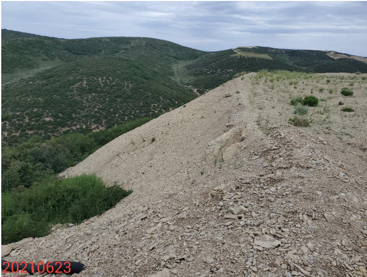
Photo 10: Photo taken from the west end of the Location, facing north. Photos show BMPs to protect and stabilize the slopes of the Location remain missing or insufficient/inadequate.
