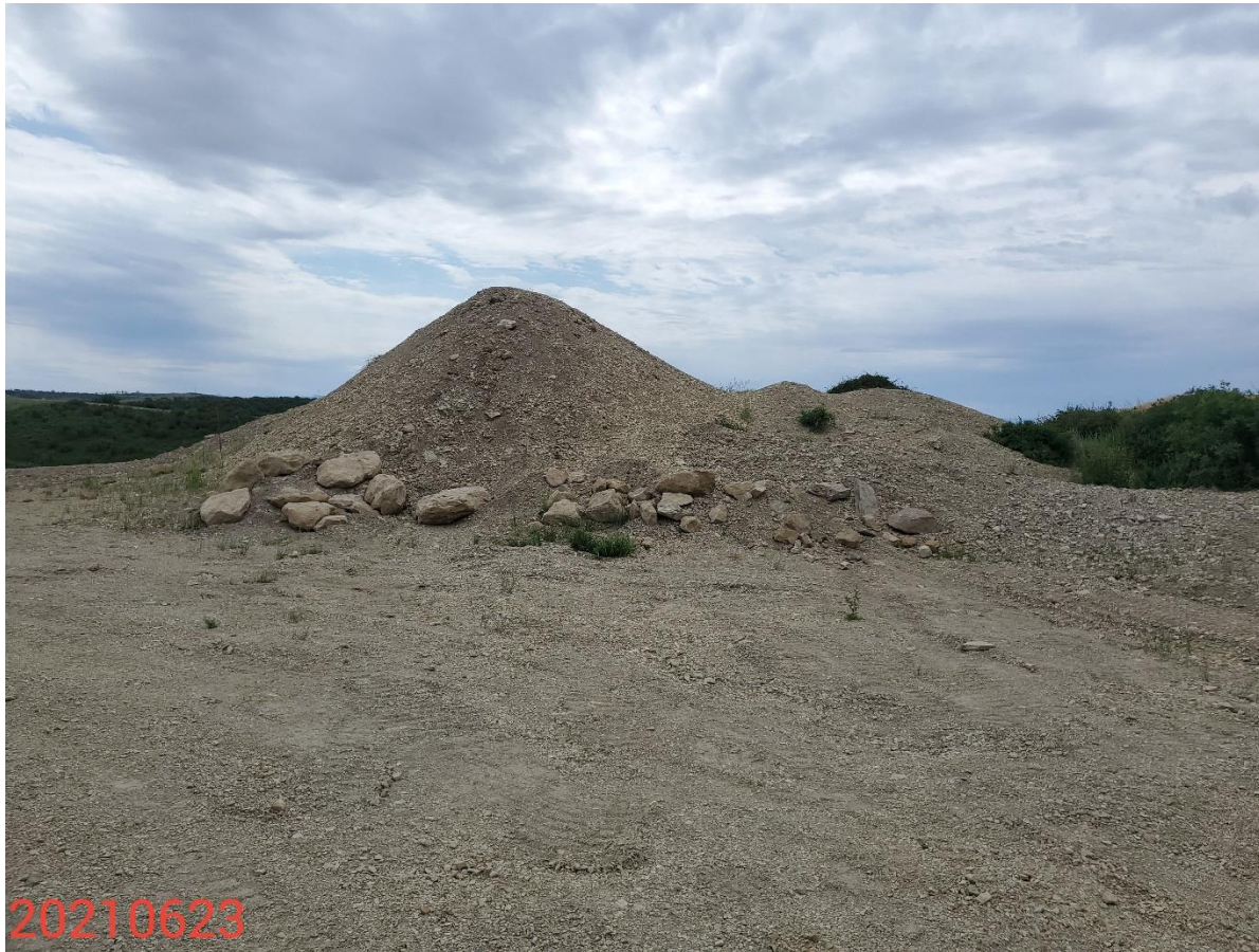
Photo 14: Photo taken from the southeast end of the Location, facing southeast. Photo shows soil stockpile. Photo also shows BMPs to protect and stabilize the slopes of the Location remain missing or insufficient/inadequate.
