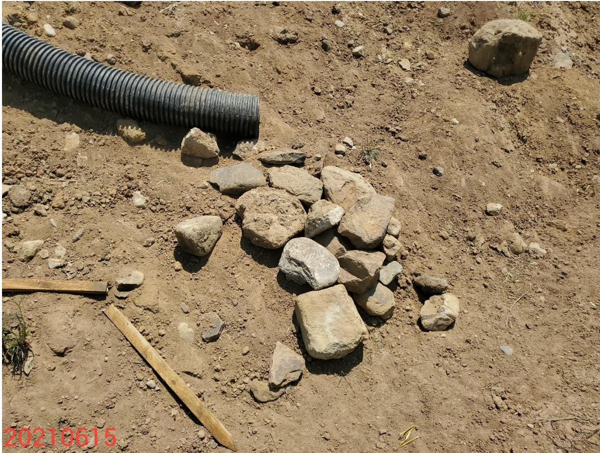
Photo 11: Continued from photo 10. Photo shows slope drain has not been properly secured, or constructed with an appropriate outlet in accordance with good engineering practice.
