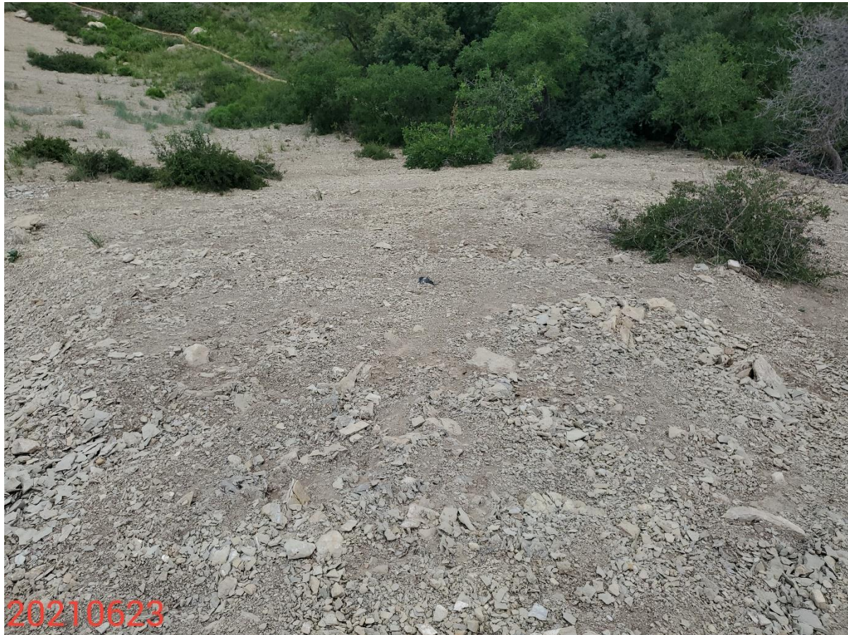
Photo 16: Photo taken from the east end of the Location, facing east. Photo shows BMPs to protect and stabilize the slopes of the Location remain missing or insufficient/inadequate.
