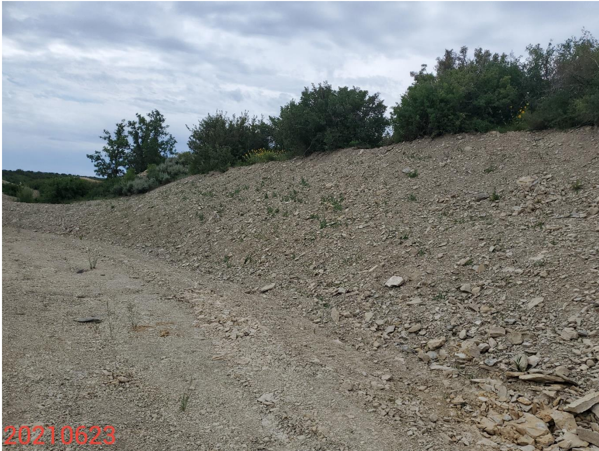
Photo 13: Photo taken from the south end of the Location, facing southeast. Photo shows BMPs to protect and stabilize the slopes of the Location remain missing or insufficient/inadequate.
