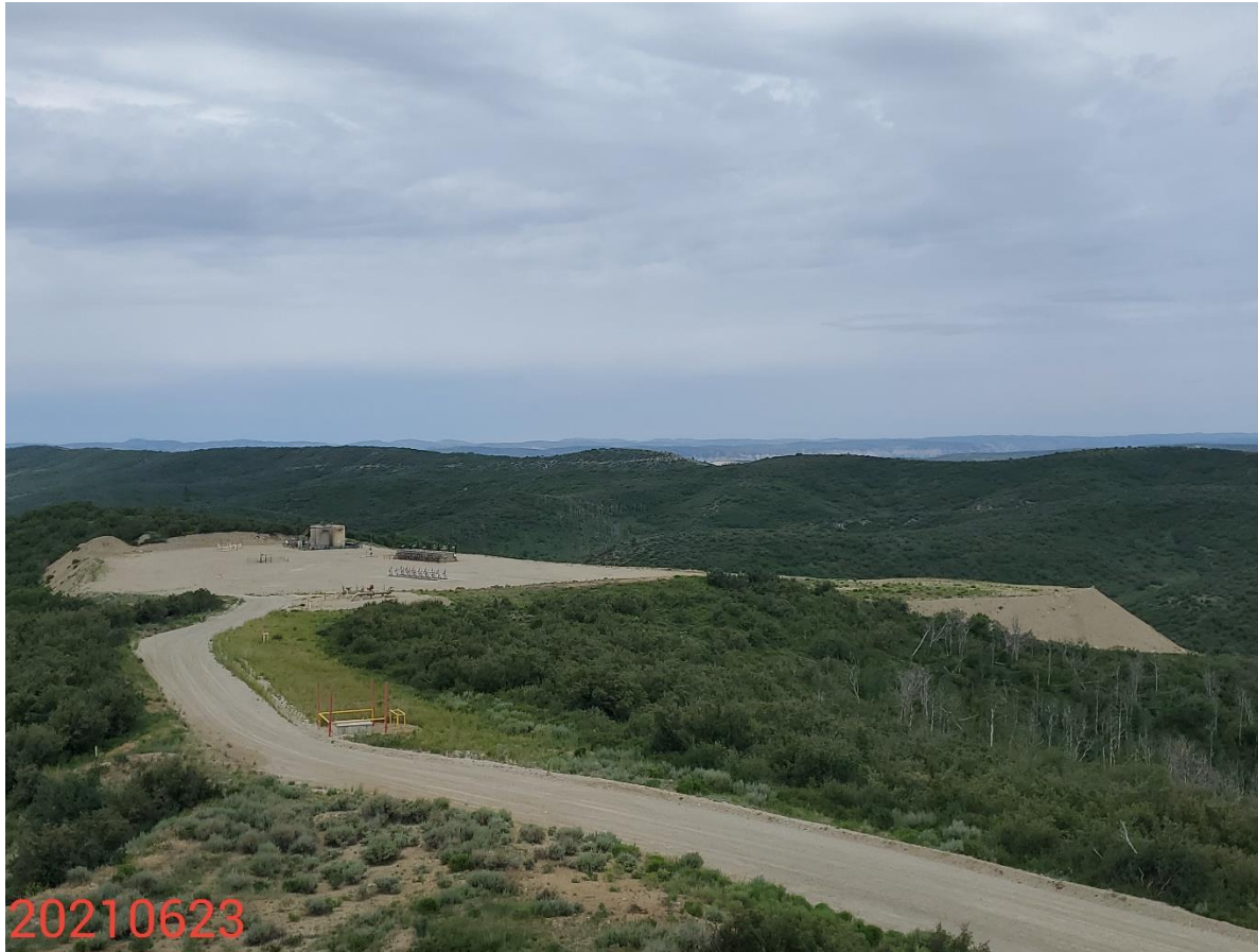
Photo 17: Photo taken northeast of the Location, facing southwest. Photo provides an overview of the Location, and shows that interim reclamation has not been performed in accordance with 1003 Rules. See photo 1 for aerial image of the Location.
