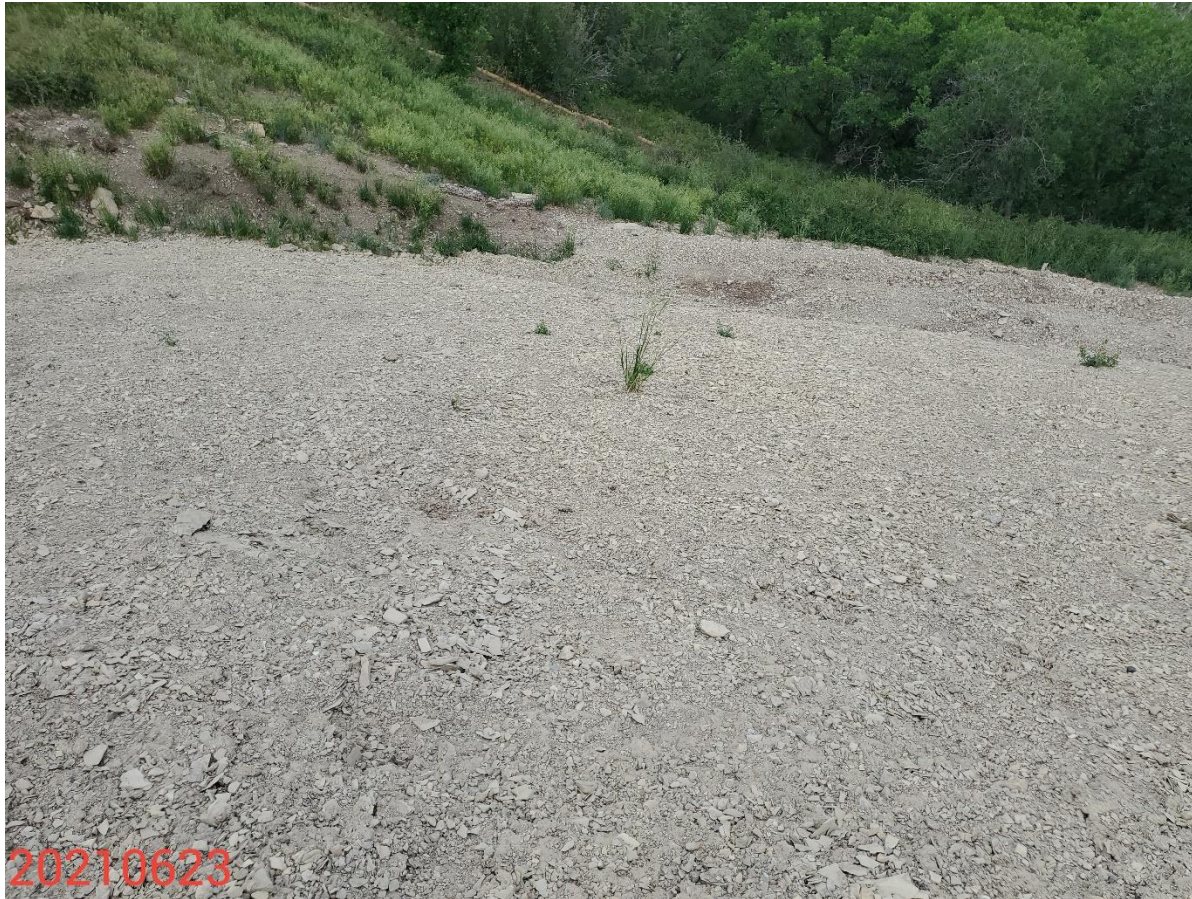
Photo 12: Photo taken from the west end of the Location, facing west. Photo shows BMPs to protect and stabilize the slopes of the Location remain missing or insufficient/inadequate.
