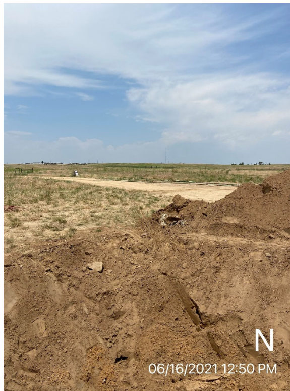
Wardell H 19-32 Wellhead Excavation
