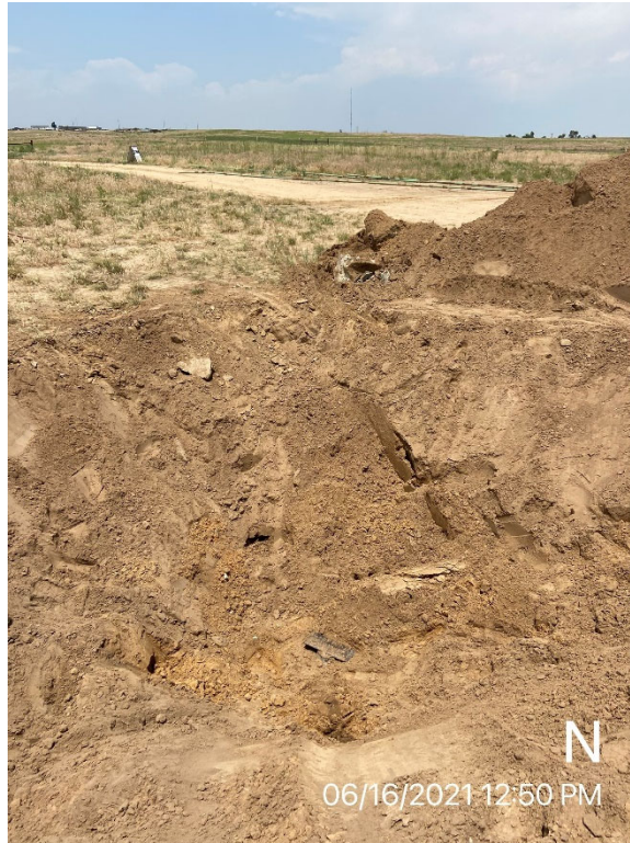
Wardell H 19-32 Wellhead Excavation (Close Up)
