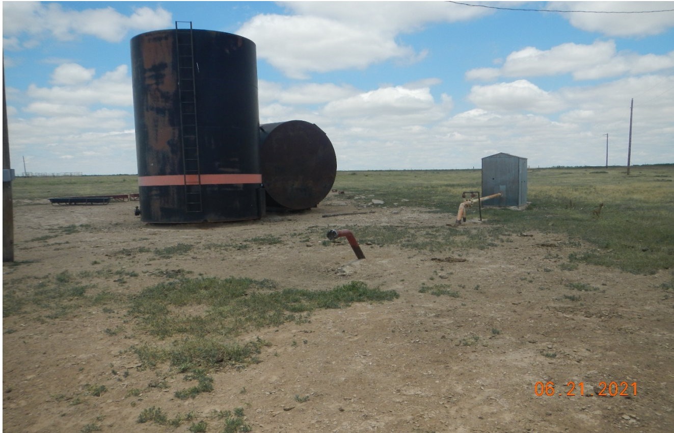
Photo 2. There are two tanks, pipe riser, and meter run that remain. All equipment should have been removed within 3 months of well abandonment.
