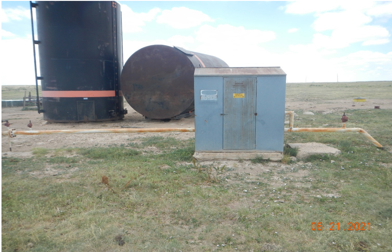
Photo 3. The meter run and shed remain at the location. All equipment should have been removed within 3 months of well abandonment.
