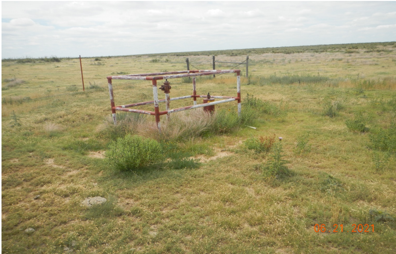
Photo 4. There is another pipeline riser that remains at the location that has not been removed.
