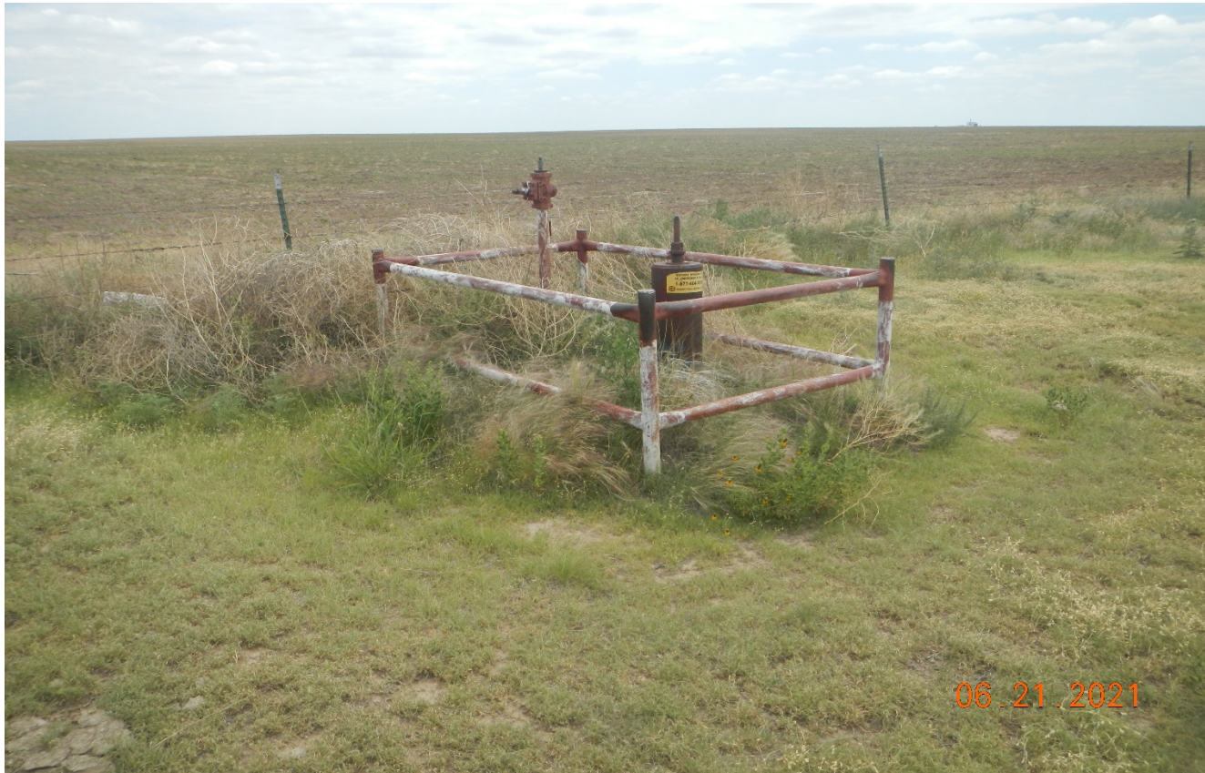
Photo 1. Approximately 100' northeast of the location is an abandoned pipeline iser which must be removed.
