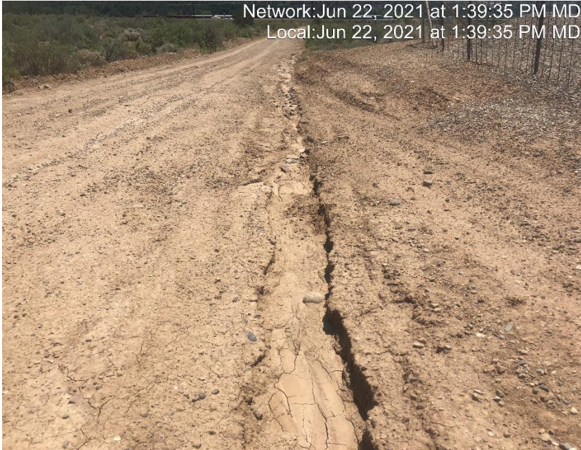
Photo #4140 No velocity checks located in ditches.
