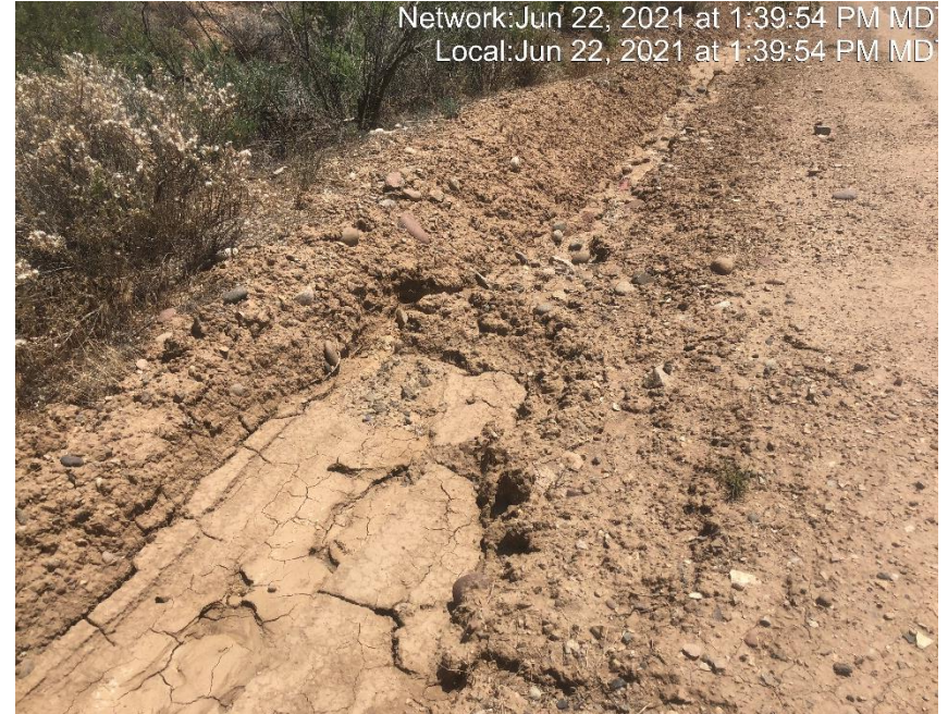
Photo #4141 No velocity checks located in ditches.
