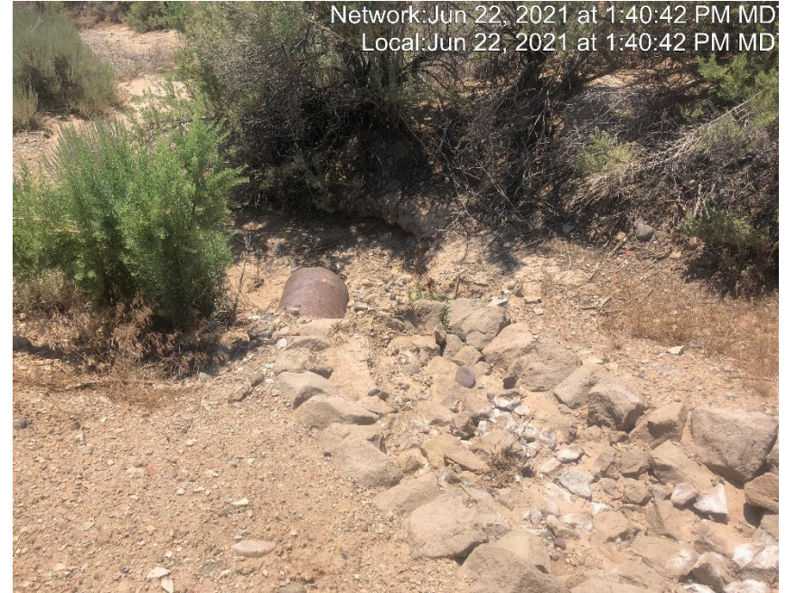
Photo #4144 Sediment trap insufficient.
