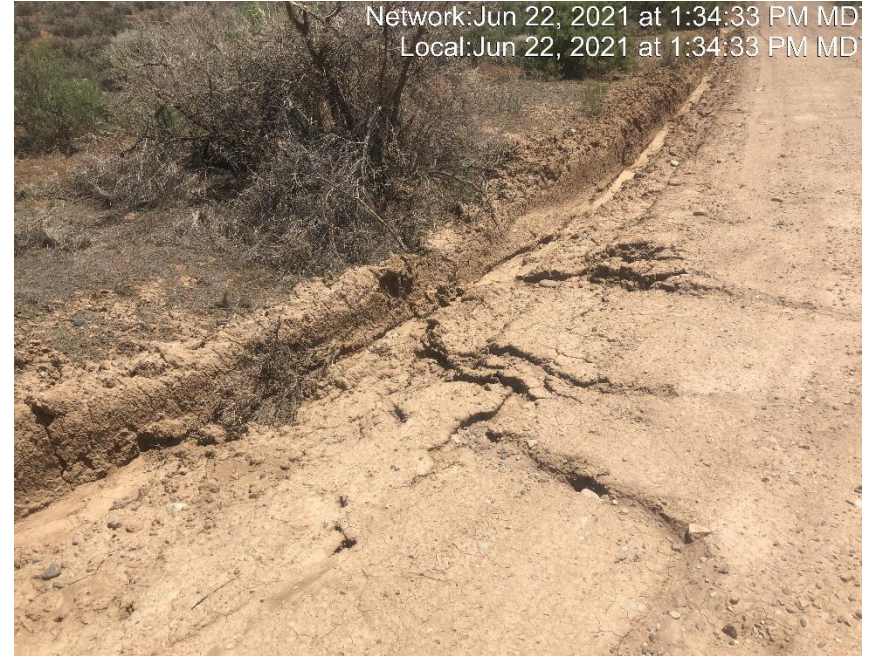
Photo #4138 Multiple places with Rill erosion occurring on location.
