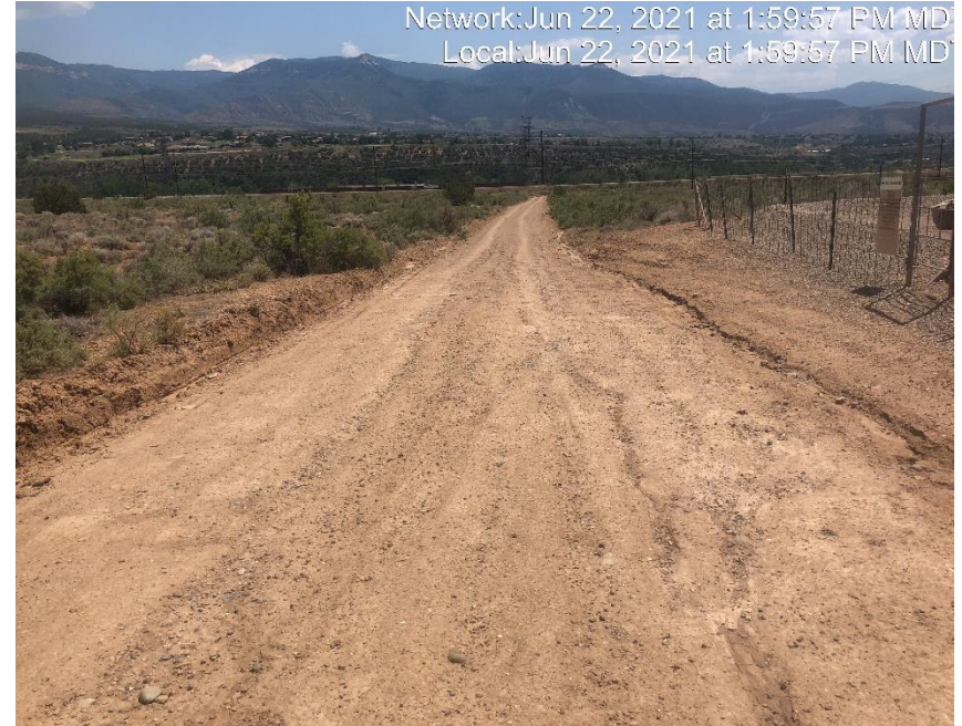
Photo #4147 No form of tracking BMP Located at entrance to location.
