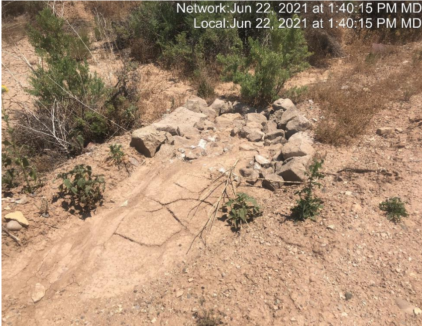
Photo #4142 Sediment trap insufficient.
