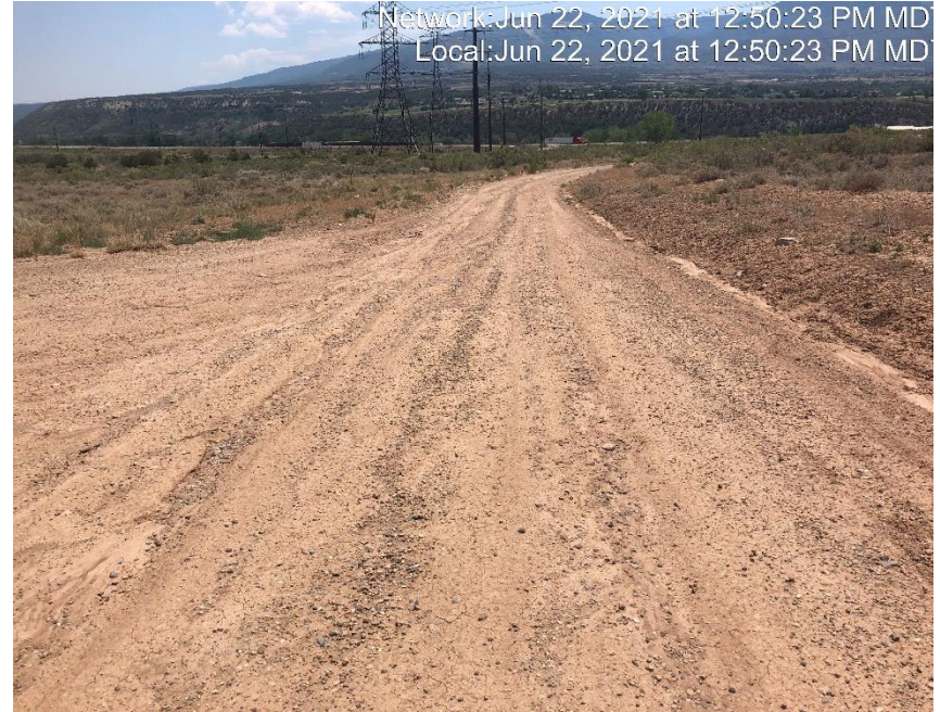
Photo #4134 No form of tracking BMP located at entrance to location.
