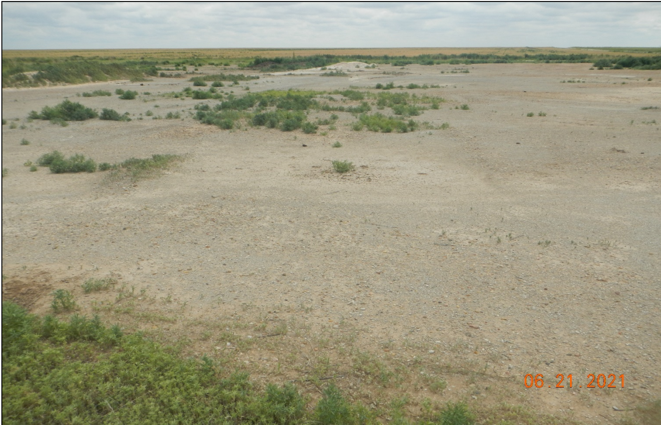
Photo 2. Facing northeast at the location. Soils are compacted and the location has not been reclaimed. Previous corrective actions were not performed. Soils must be decompacted by cross ripping to a depth of 18 inches.
