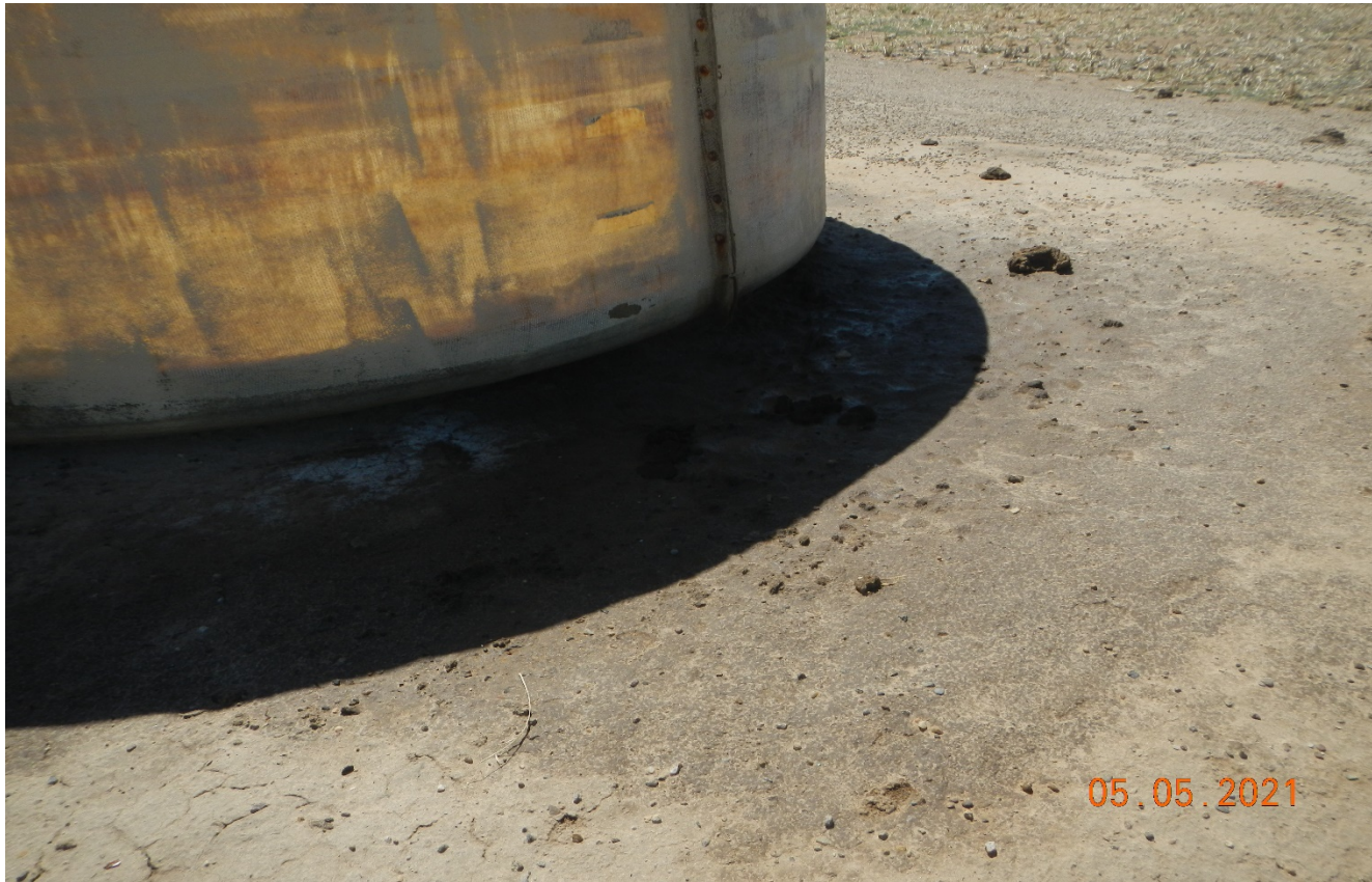
Photo 3. There appears to have been a leak at the tank due to stained soil in this area. If tank contains produced salty water, this can impact the soil and crop growth.
