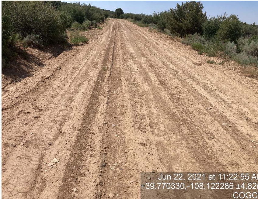
Lack of stabilization/compaction/erosion
