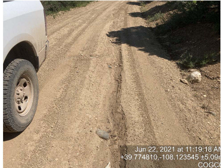
Lack of stabilization/compaction/erosion
