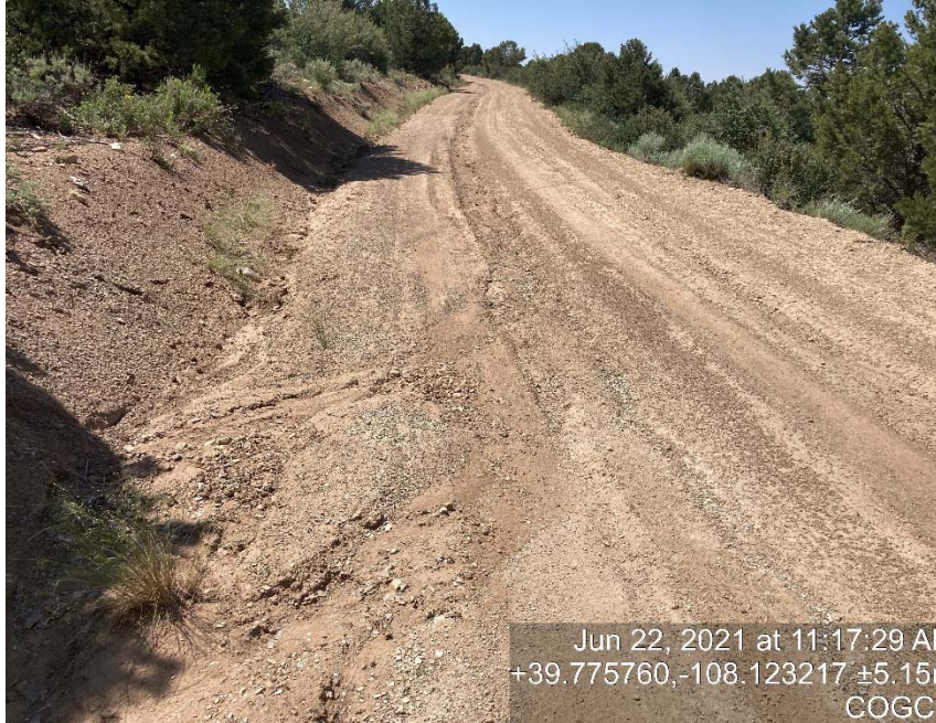
Lack of stabilization/compaction/erosion
