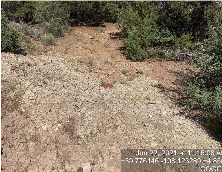
One of the sediment traps along access road
