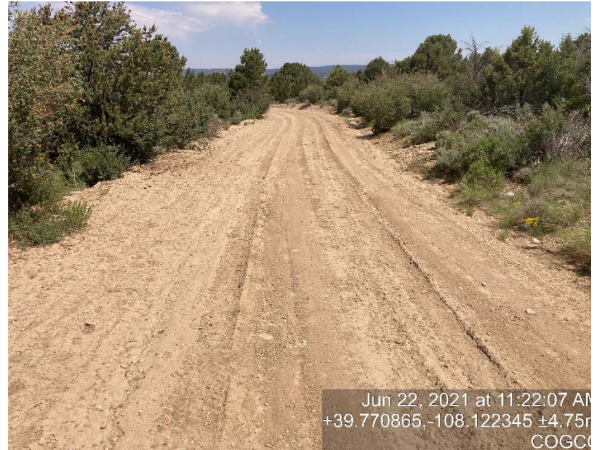
Lack of stabilization/compaction/erosion
