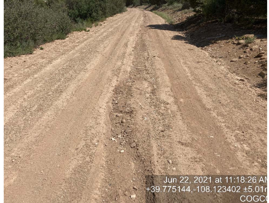
Lack of stabilization/compaction/erosion
