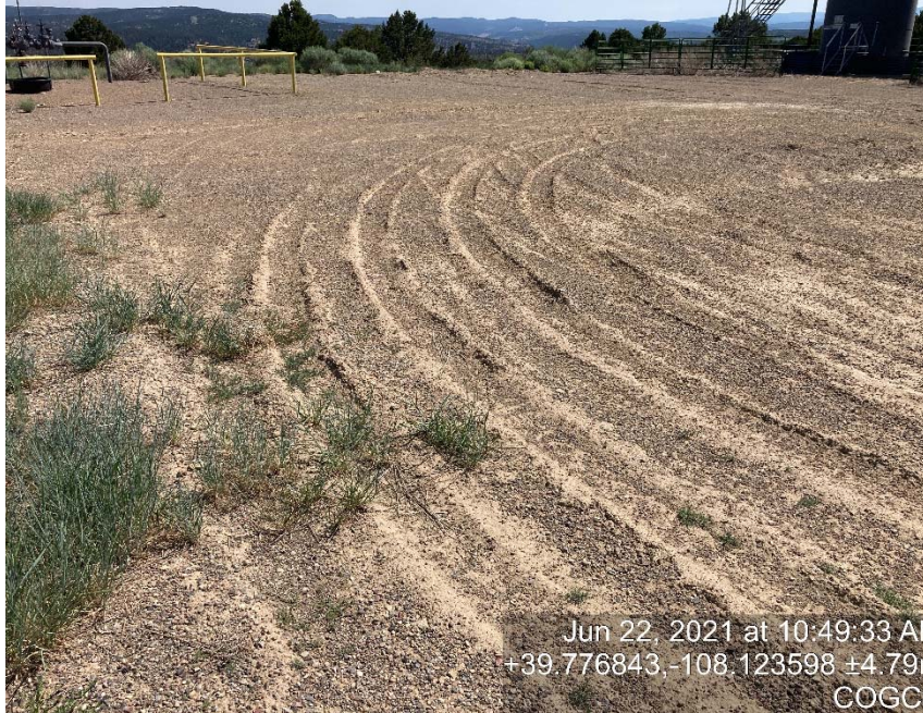
Lack of stabilization/compaction
