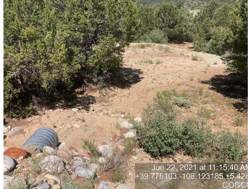
One of the sediment traps along access road
