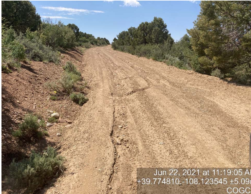
Lack of stabilization/compaction/erosion
