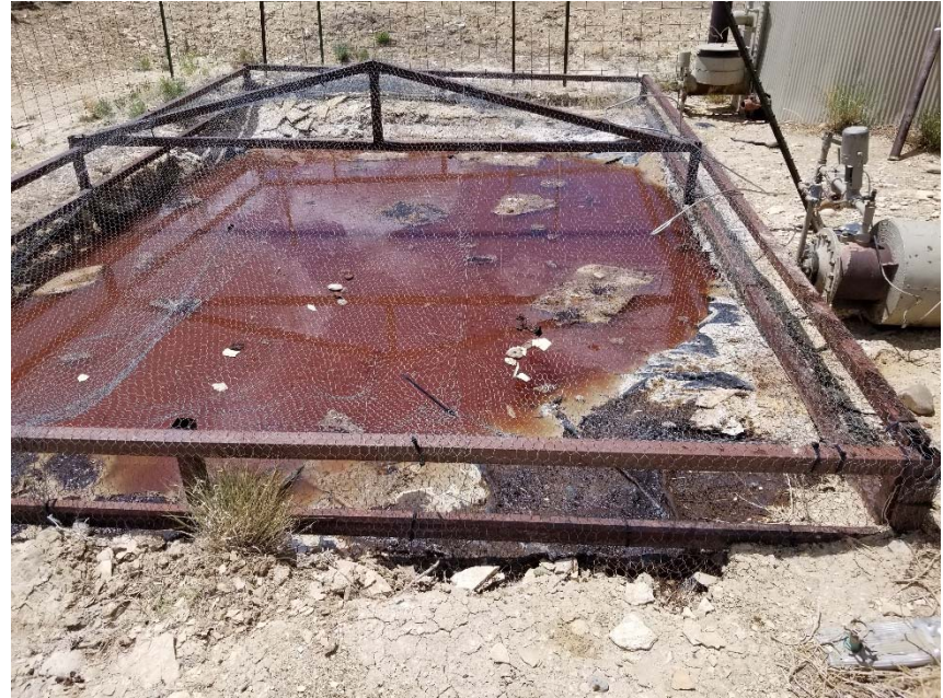
Photo 5. Pit without permit. Less than 2 feet of freeboard and oil on pit.
