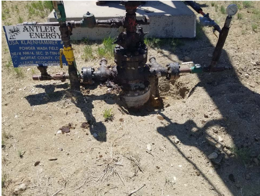
Photo 2. Stained soil at wellhead.
