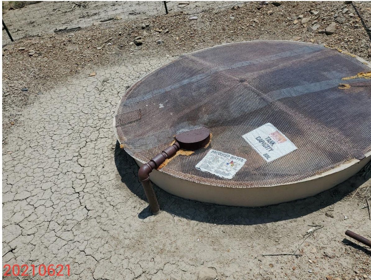
Photo 3: Photo shows produced water tank. Tank capacity no longer identified.
