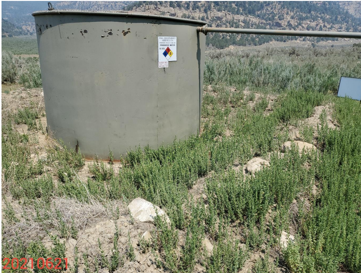
Photo 4: Photo shows weed weed/plant establishment on and within the secondary containment BMP. Containment BMP also does not appear to be sufficient in size to contain 150% volume of the tank.
