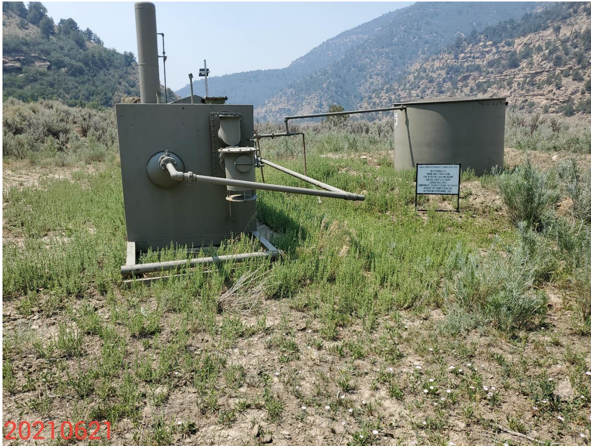
Photo 3: Photo shows weed/plant establishment at the separator and tank.
