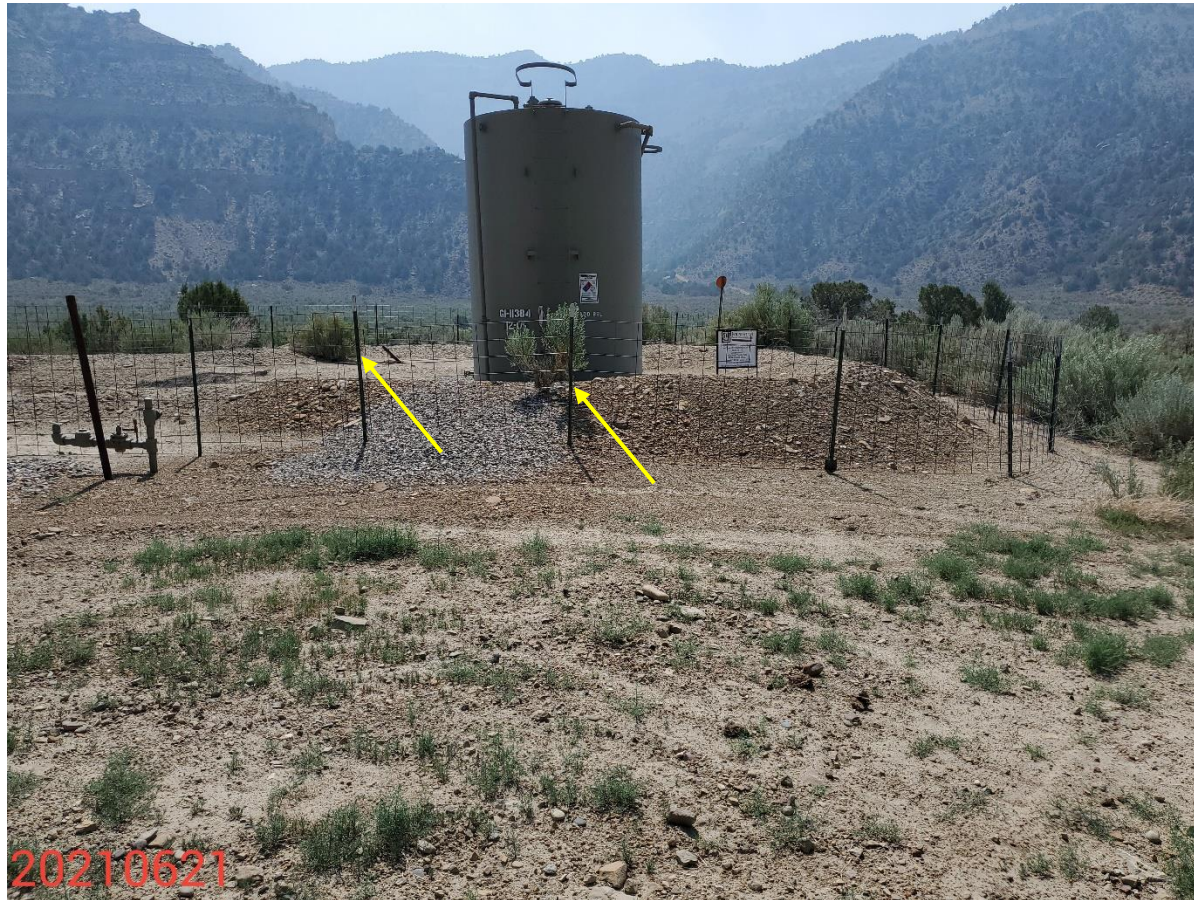
Photo 3: Photo taken from the south end of the Location, facing east. Photo shows example of vegetation observed established on, and within the secondary containment BMP; vegetation establishment compromises the integrity and permeability of the containment BMP.
