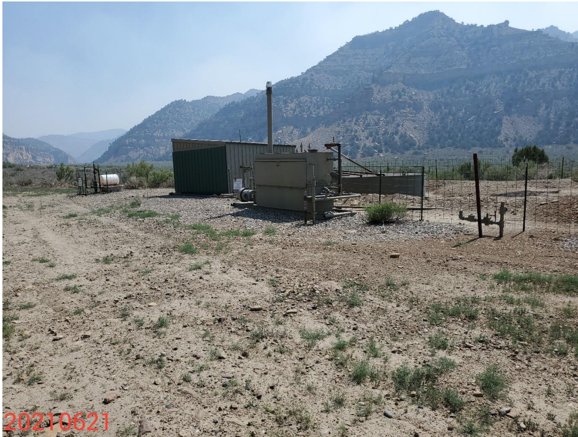
Photo 2: Photo taken from the south end of the Location, facing west. Photo shows compressor/separator/produced water tank equipment.
