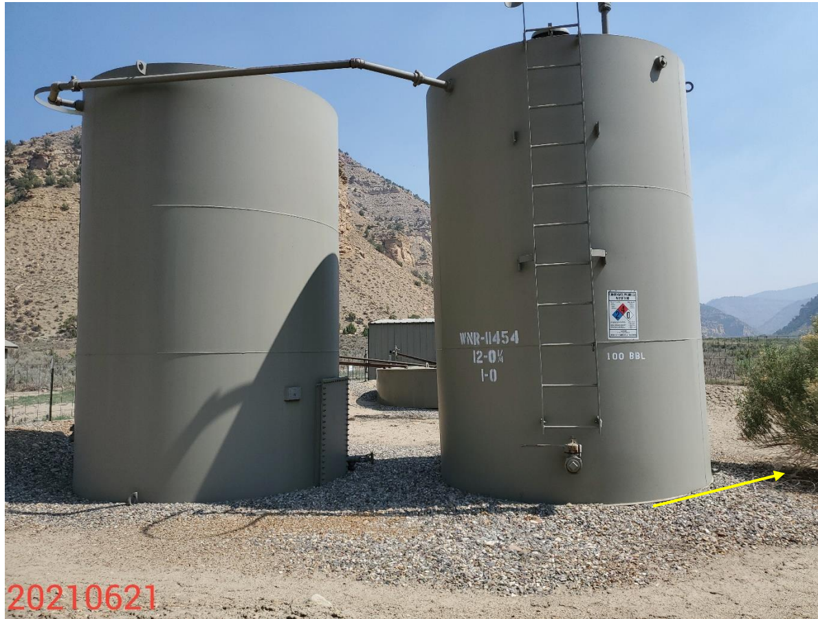
Photo 7: Photo of the tank battery on the southeast end of the Location. Photo also shows example of vegetation observed established on, and within the secondary containment BMP; vegetation establishment compromises the integrity and permeability of the containment BMP.
