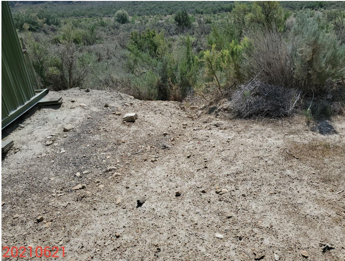
Photo 5: Photo taken from the east end of the Location, facing east. Photo shows areas where stormwater runoff concentrates and discharges from the pad.
