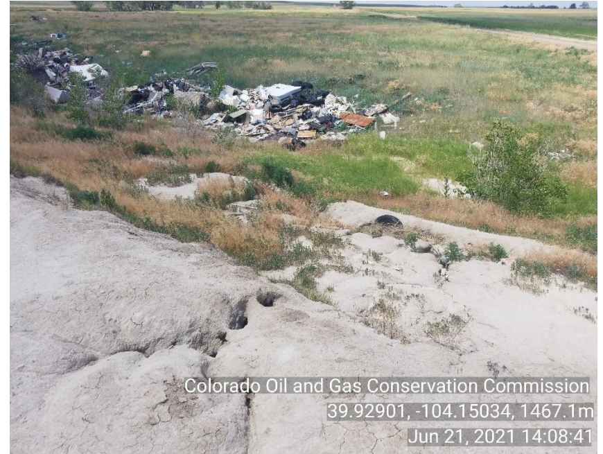
Photo 12 pit berm sediment running into drainage.
