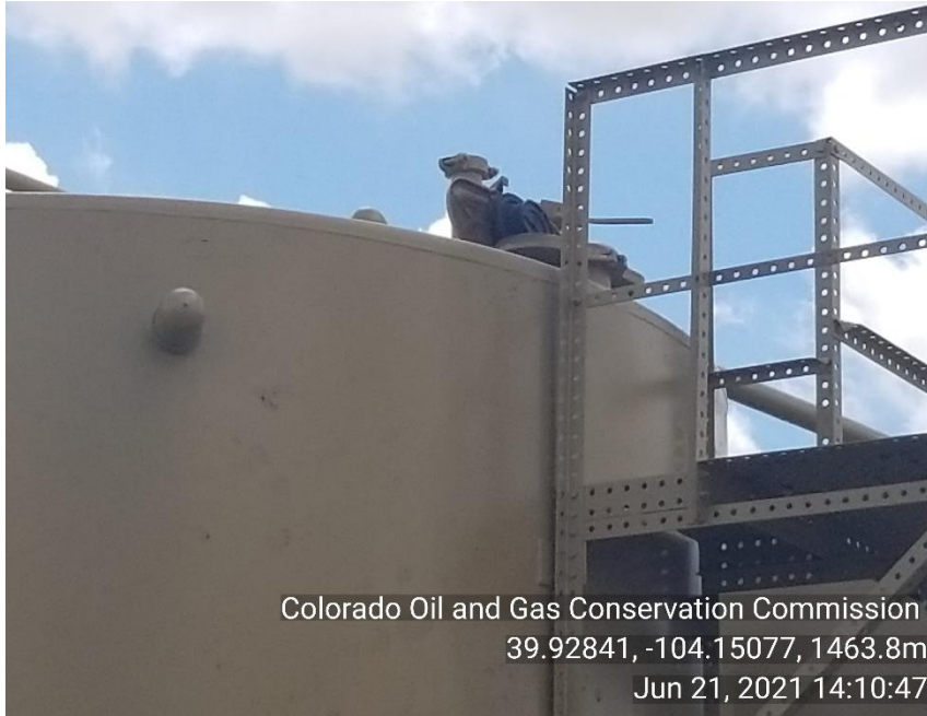
Photo 17 gauge hatch open on crude oil tank.
