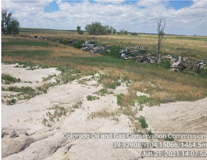
Photo 11 no BMP in place to prevent pit berm sediment from leaving location.
