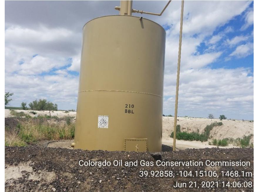
Photo 8 Produced water tank NFPA placard faded need to be replaced.
