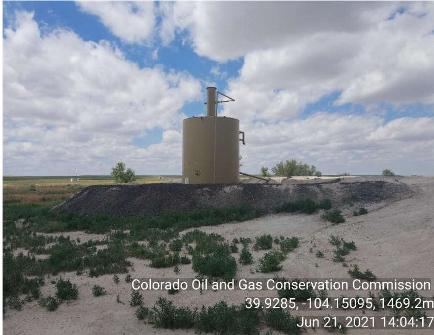
Photo 5 Produced water tank.
