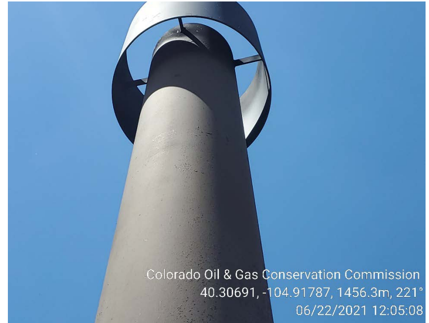
Heater treater burner stack
