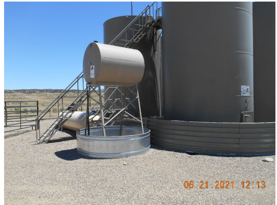
Methanol tank with secondary containment.
