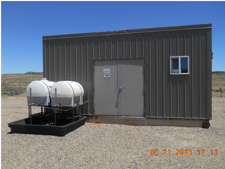
Pump housing. Chemical drums with secondary containment.
