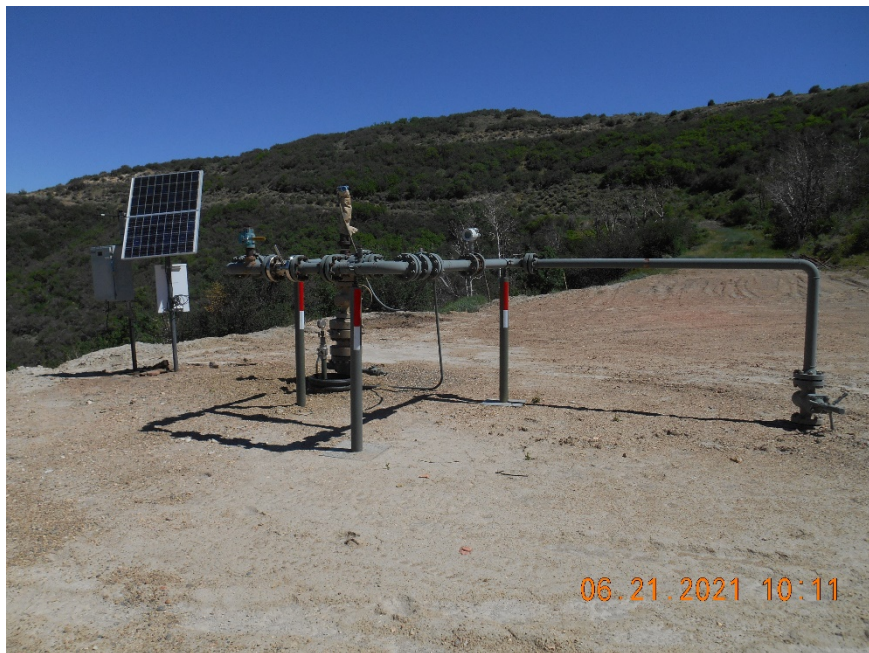
Injection wellhead
