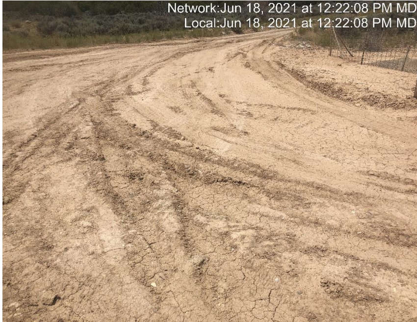
Photo #4114 No form of tracking BMP located at the entrance to location.
