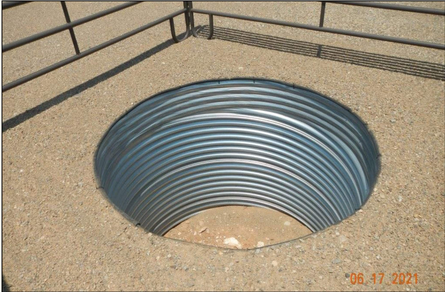
Photo 2. View of cellar that is approximately 6-feet deep observed on the well pad. This needs to be covered or wildlife escape ramp installed.
