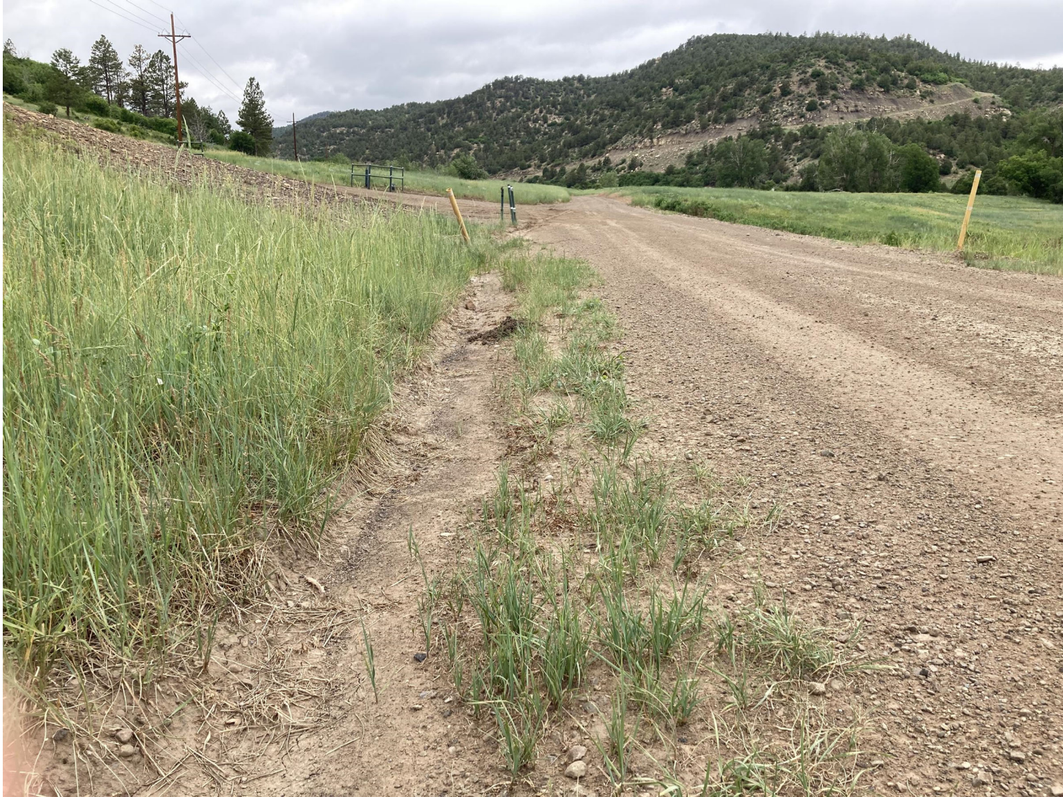
PHOTO 4: THE BAR DITCH WAS DOMINATED TO RECEIVE STORMWATER FROM THE MAIN LEASE ROAD ON SOUTH FORK.
