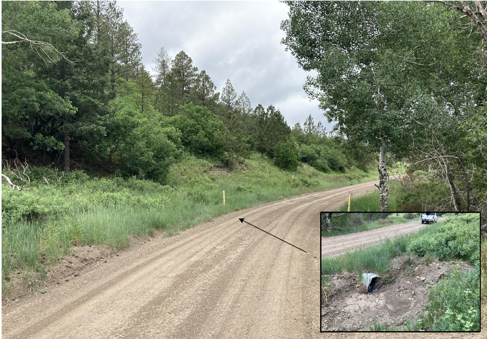
PHOTO 2: THE SEDIMENT ACCUMULATION WAS REMOVED FROM THE CULVERT INLET. THE BAR DITCH WAS DOMINATED TO RECEIVE STORMWATER AND DIRECT THE FLOW TO THE CULVERT INLET. THE SEDIMENT ACCUMULATION WAS REMOVED FROM THE CULVERT INLET.
