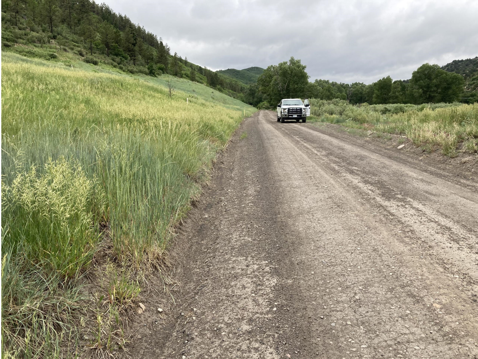
PHOTO 1: THE SEDIMENT ACCUMULATION WAS REMOVED FROM THE BAR DITCH AND THE DITCH WAS DOMINATED TO RECEIVE STORMWATER.
