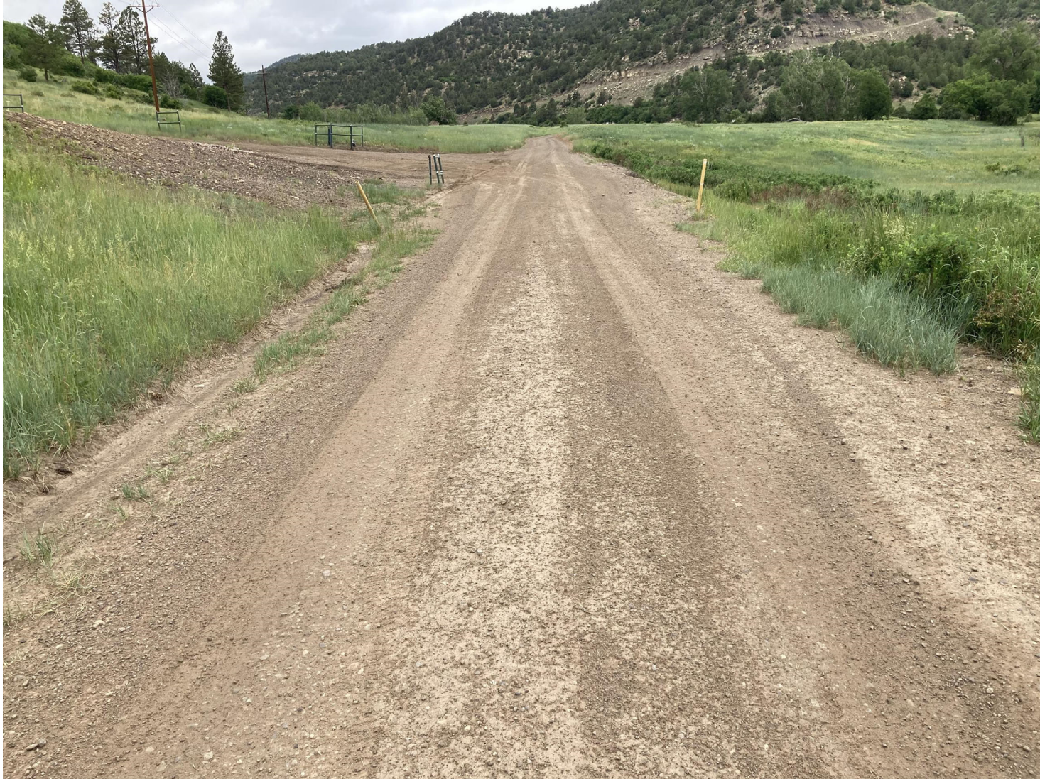
PHOTO 3: THE BAR DITCH WAS DOMINATED TO RECEIVE STORMWATER AND DIRECT THE FLOW TOWARD THE CULVERT INLET. THE LEASE ROAD WAS CROWNED TO ESTABLISH SHEET FLOW OFF OF THE ROAD SURFACE AND ELIMINATE THE TIRE RUTS.
