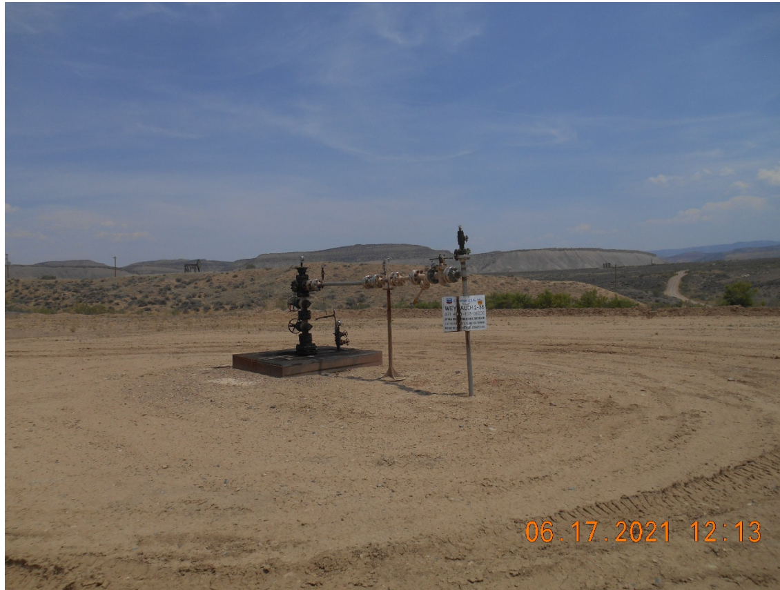
Injection Wellhead
