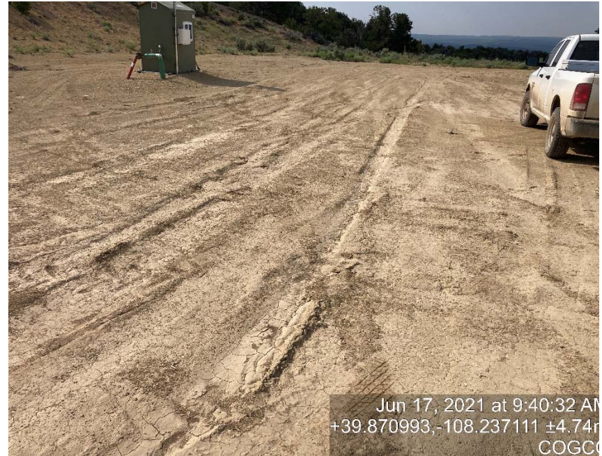
Lack of stabilization/compaction
