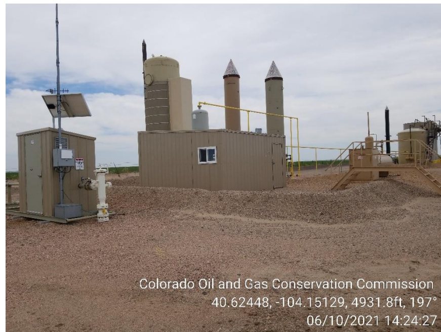
Photo 4 – Heater Treater and ECDs
