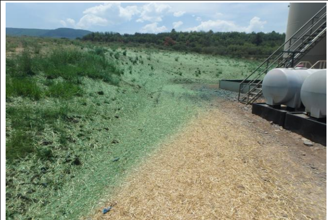
My Way Ranch 17-7 after Mulching and Tackifying Cut Slope
