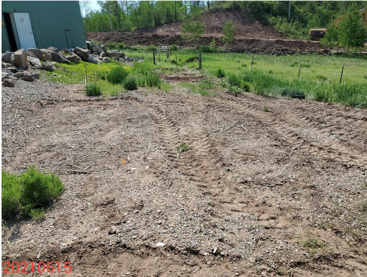
Photo 14: Photo shows that neither a sediment pond/trap BMP has been installed, or reclamation conducted on the southern areas of the Location.
