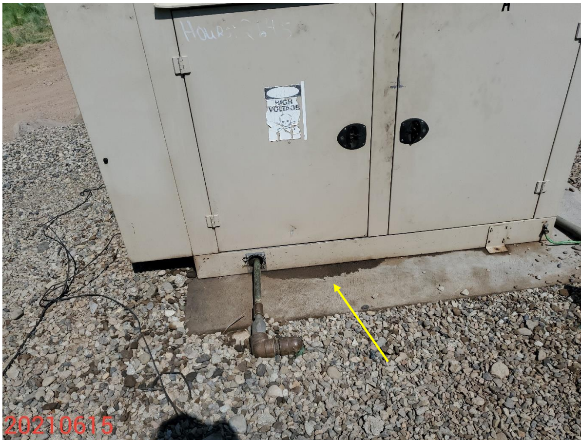
Photo 2: Continued from photo 1. Photo shows mechanical issues appear to remain an issue for the equipment, as additional fluids can be observed leaking at the base (arrow).
