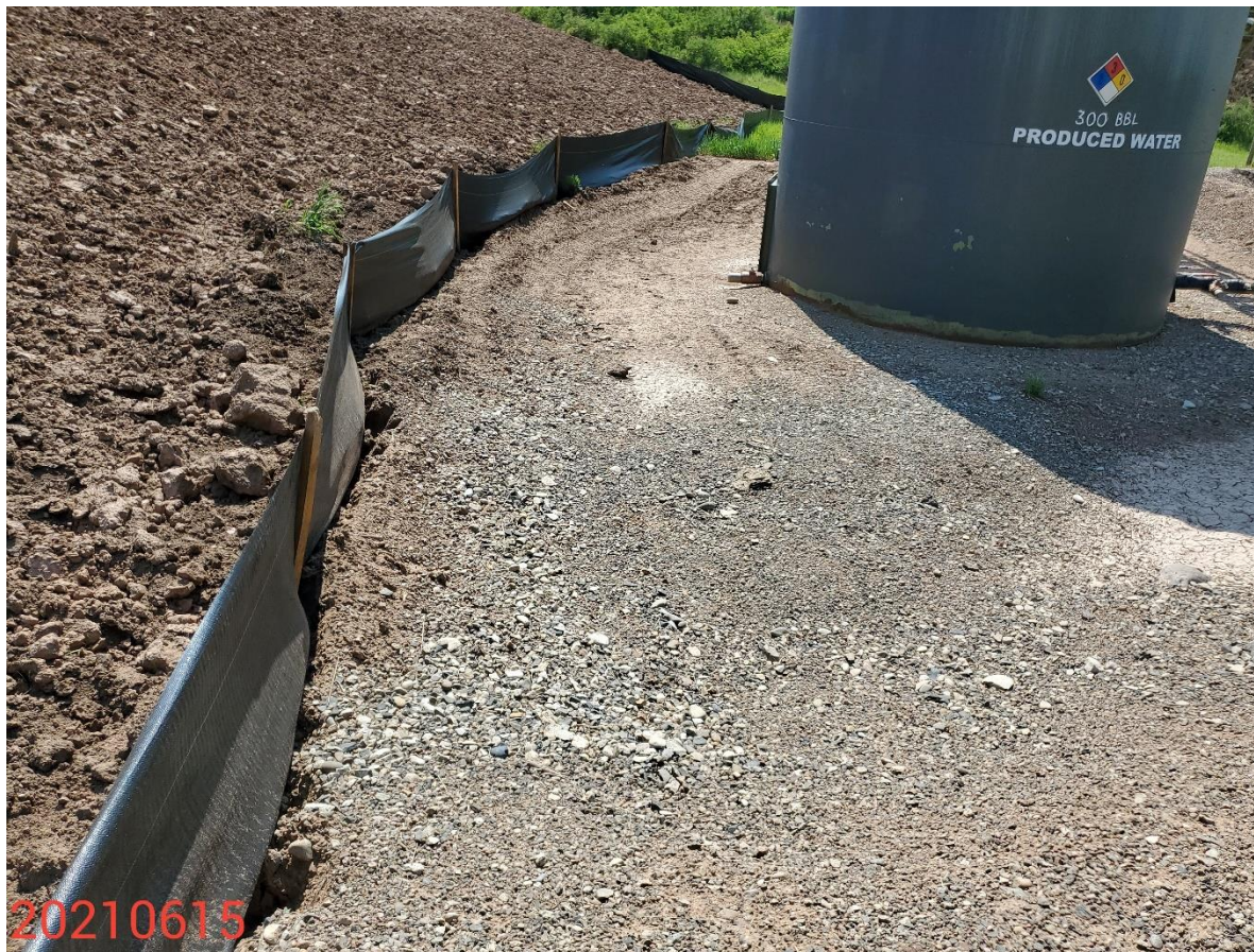
Photo 8: Previous inspection observed that the containment BMP at the tanks was inadequate. Photo shows that BMP appears to remain inadequate in accordance with Rule 603.o
