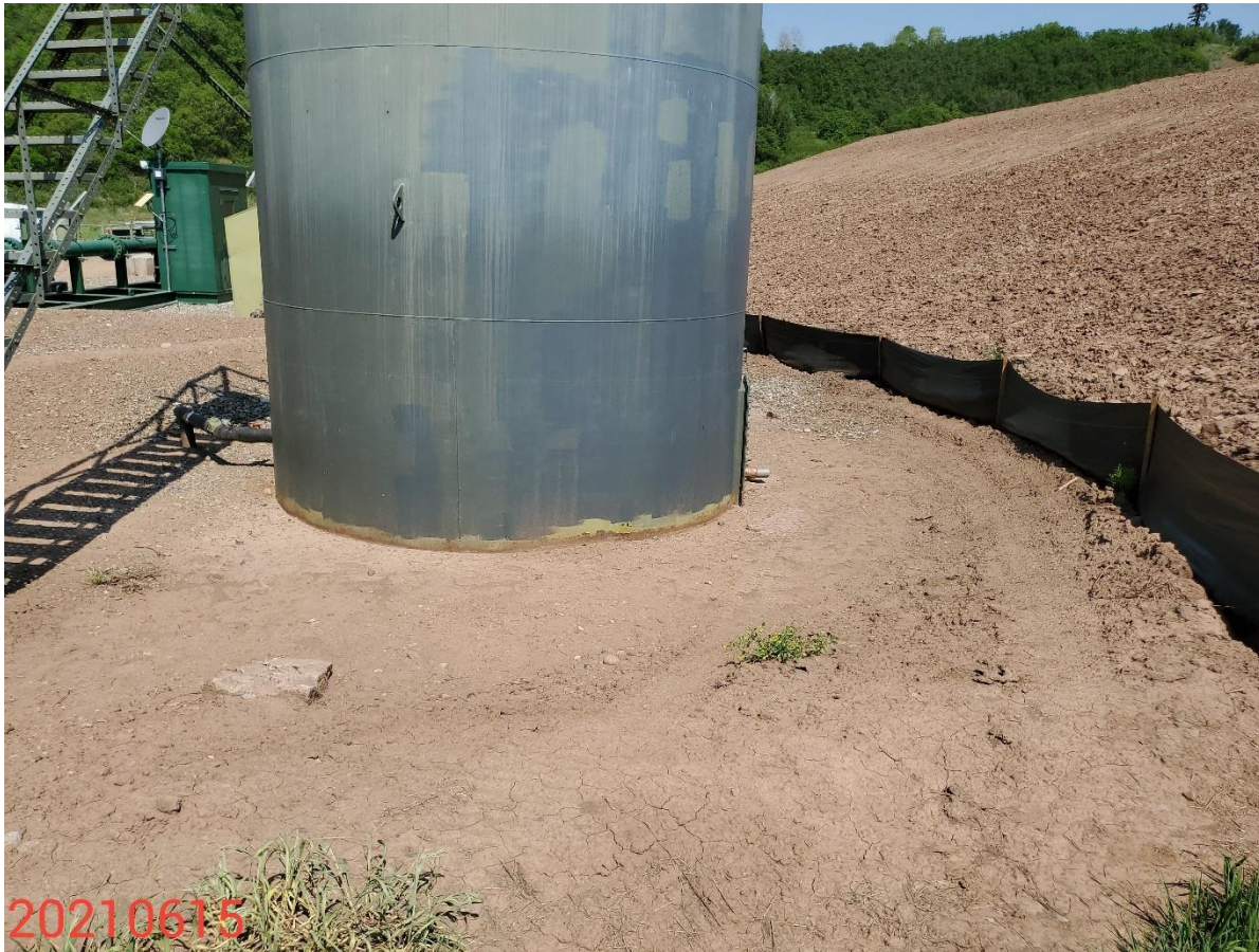
Photo 10: Previous inspection observed that the containment BMP at the tanks was inadequate. Photo shows that BMP appears to remain inadequate in accordance with Rule 603.o
