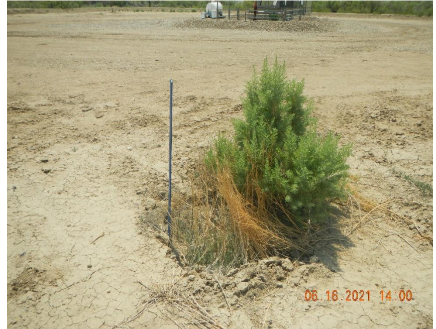
Subsidence of ground at buried line marker.
