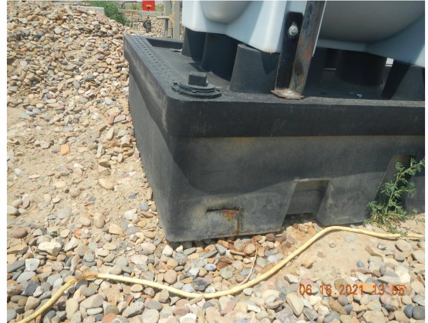
Damaged secondary container.
