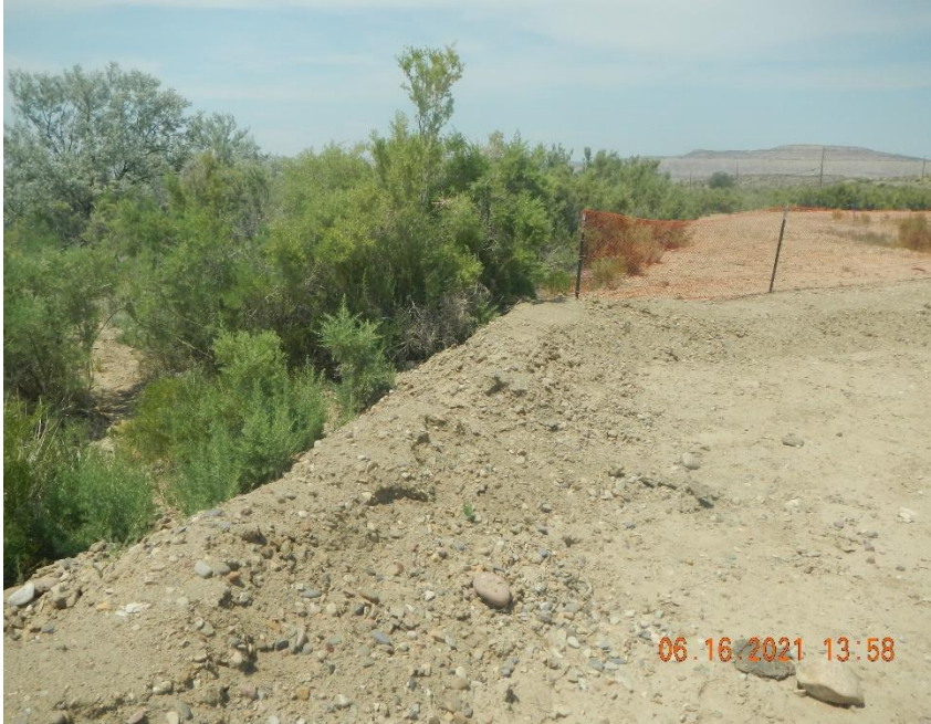
Damaged perimeter berm.
