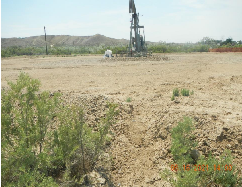
Damaged perimeter berm.
