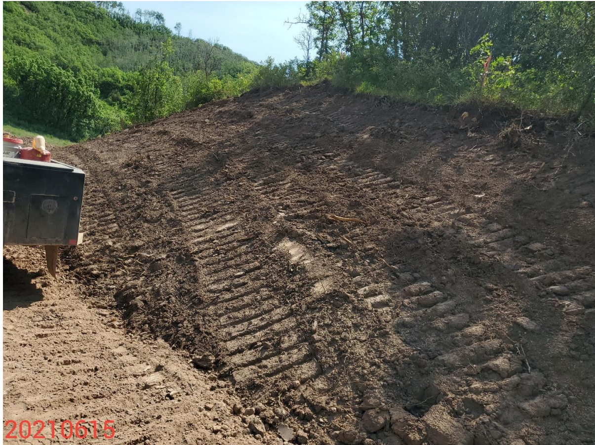
Photo 16: Photo taken from the cut slopes on the south end of the Location, facing east. Photo shows control measures to protect and stabilize the cut slopes are missing or insufficient.
