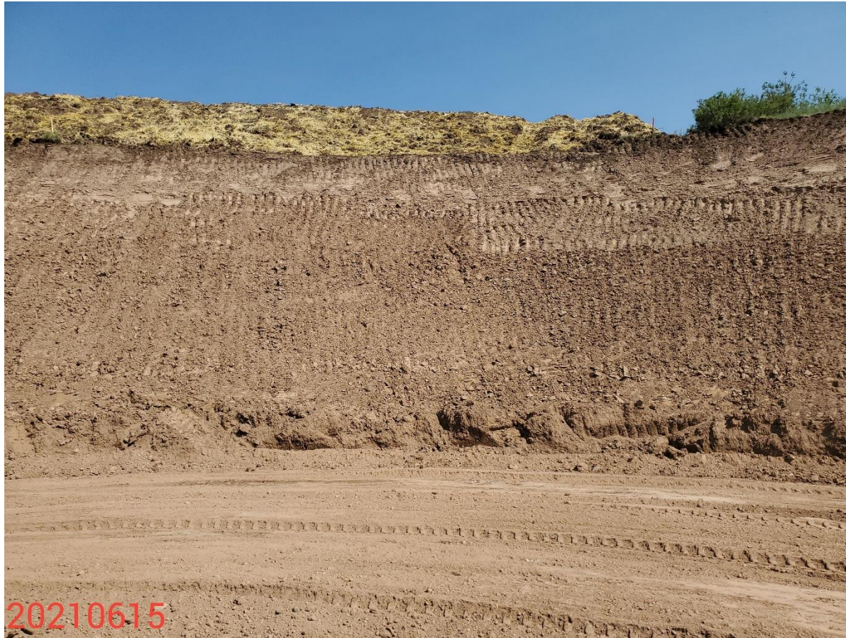
Photo 11: Photo shows the cut slope on the north end of the Location, facing northeast. Photo shows control measures to protect and stabilize the cut slopes are missing or insufficient. It appears Operator implemented tracking along slopes; tracking insufficient and was not applied up and down the slope per good engineering practices.
