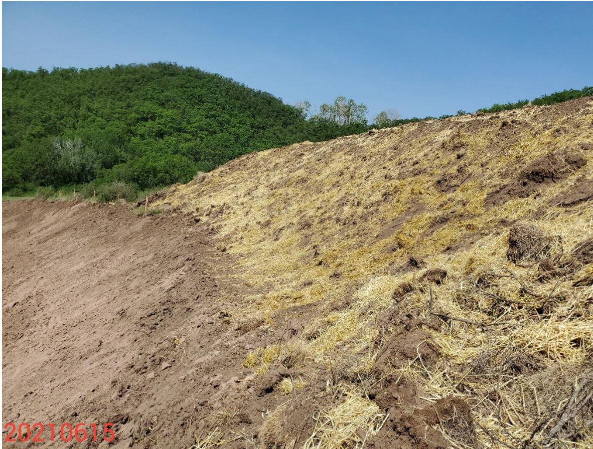
Photo 8: Continued from photo 7. Photo shows perimeter stormwater controls to mitigate sediment transport from the topsoil stockpile is missing on the southern/western ends of the topsoil stockpile
