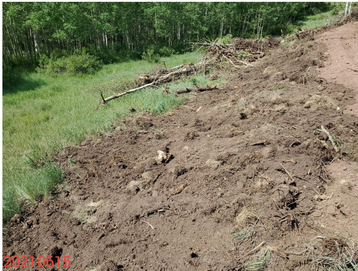
Photo 23: Continued from photo 22. Photo shows Stormwater erosion control BMPs to prevent off site sediment transport, and to stabilize the slopes along the access road remain missing or insufficient.
