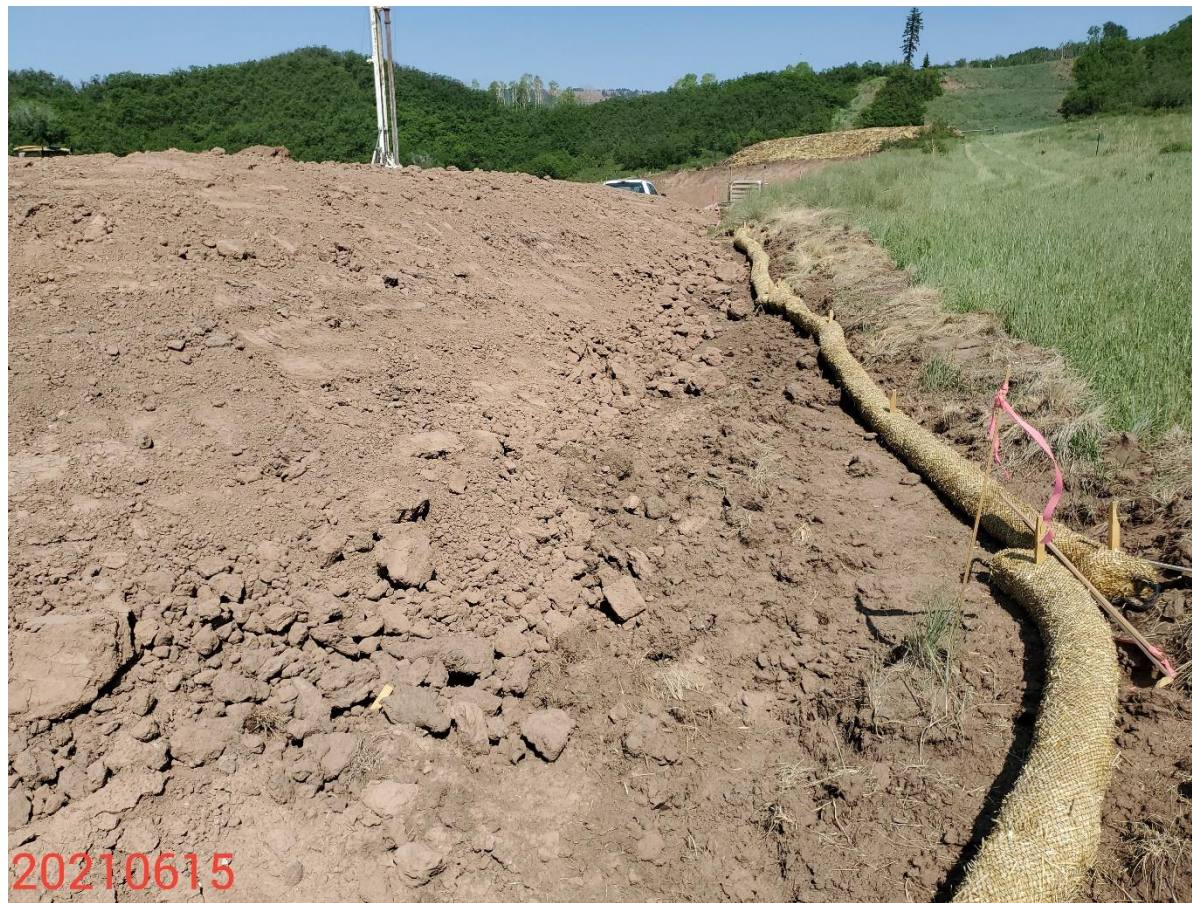
Photo 20: Photo taken from the southeast end of the Location, facing north. Photo shows perimeter stormwater control measures are missing or insufficient at Location perimeter and access road entrance. Photo also shows control measures to protect and stabilize the slopes are missing or insufficient. Wattles have not been installed in accordance with good engineering practices.
