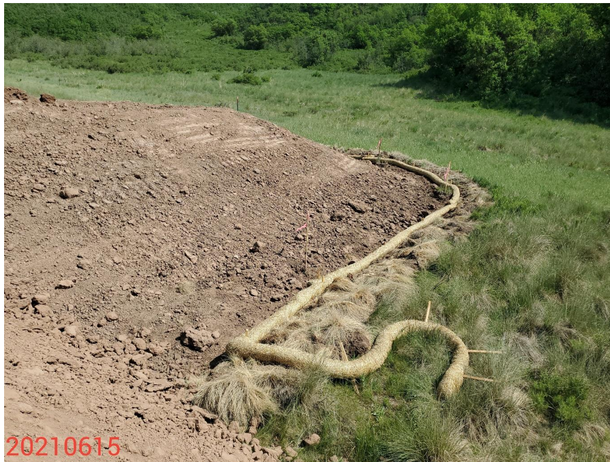
Photo 19: Photo taken from the south end of the Location, facing east. Photo shows perimeter stormwater control measures are missing or insufficient at Location perimeter and entrance. Photo also shows control measures to protect and stabilize the slopes are missing or insufficient.
