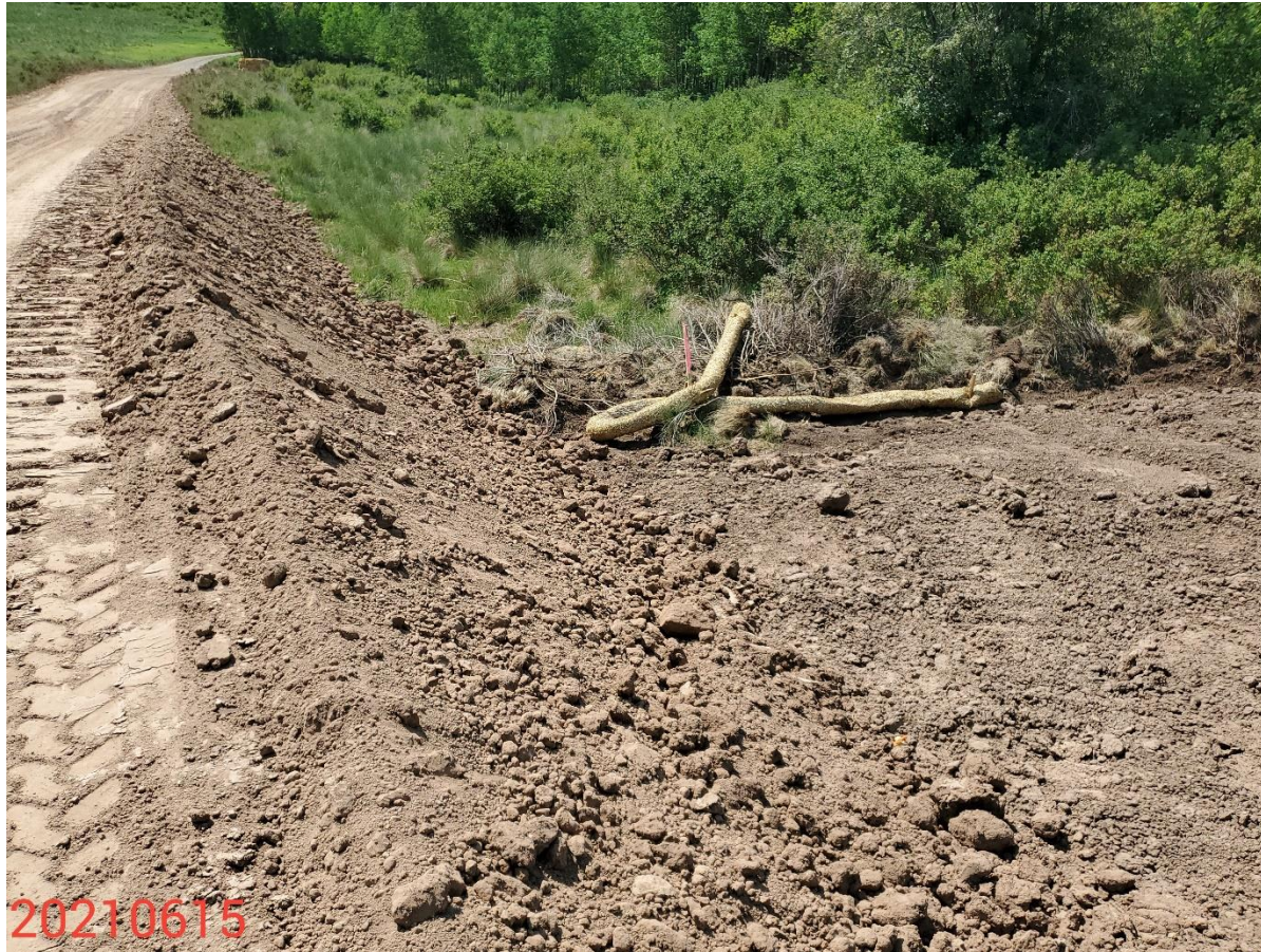
Photo 18: Photo taken from the south end of the Location, facing south. Photo shows perimeter stormwater control measures are missing or insufficient at Location perimeter/location entrance/access road. Photo also shows control measures to protect and stabilize the slopes are missing or insufficient.
