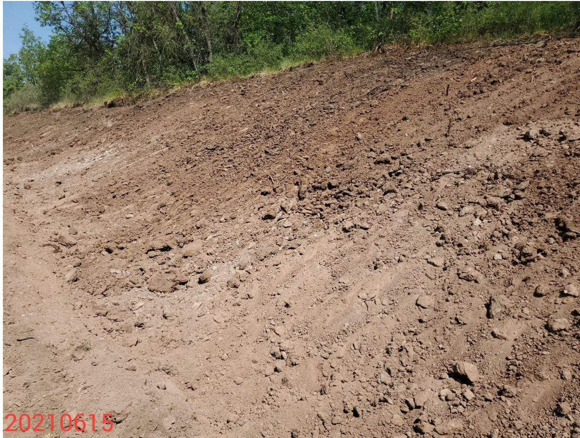
Photo 25: Photo shows control measures to protect/stabilize the cut slopes along the access road are missing or insufficient.
