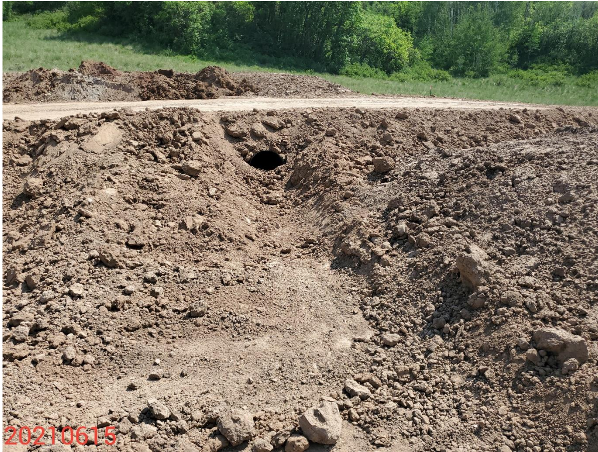
Photo 17: Photo shows culvert at the Location entrance. Sediment partially filling the inlet/outlet of culvert. Ensure culvert remains free of sediment and in proper functioning condition. .
