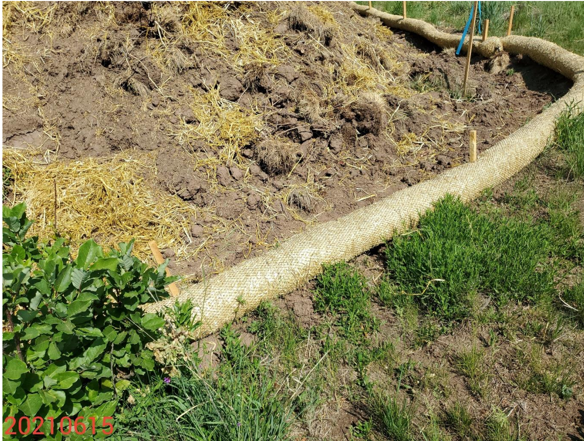
Photo 7: Continued from photo 6. Photo shows erosion logs have not been installed in accordance with good engineering practices; logs have only been placed onto the top of the soil and staked; erosion logs have not been properly trenched and backfilled.
