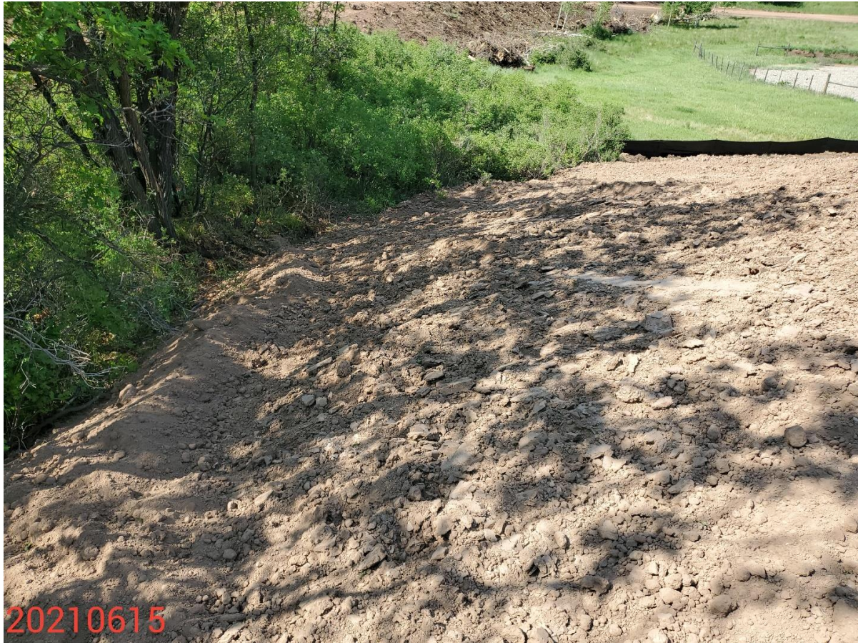
Photo 15: Photo taken from the southwest end of the Location, facing west. Photo shows control measures to protect/stabilize the slopes, and perimeter control measures to allow for sediment laden-free stormwater discharge are missing or insufficient.
