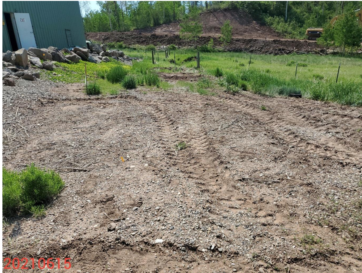
Photo 29: Photo shows areas west of the Location identified within the location drawing where a sediment pond was planned to be constructed. Photo shows BMP has not been constructed.
