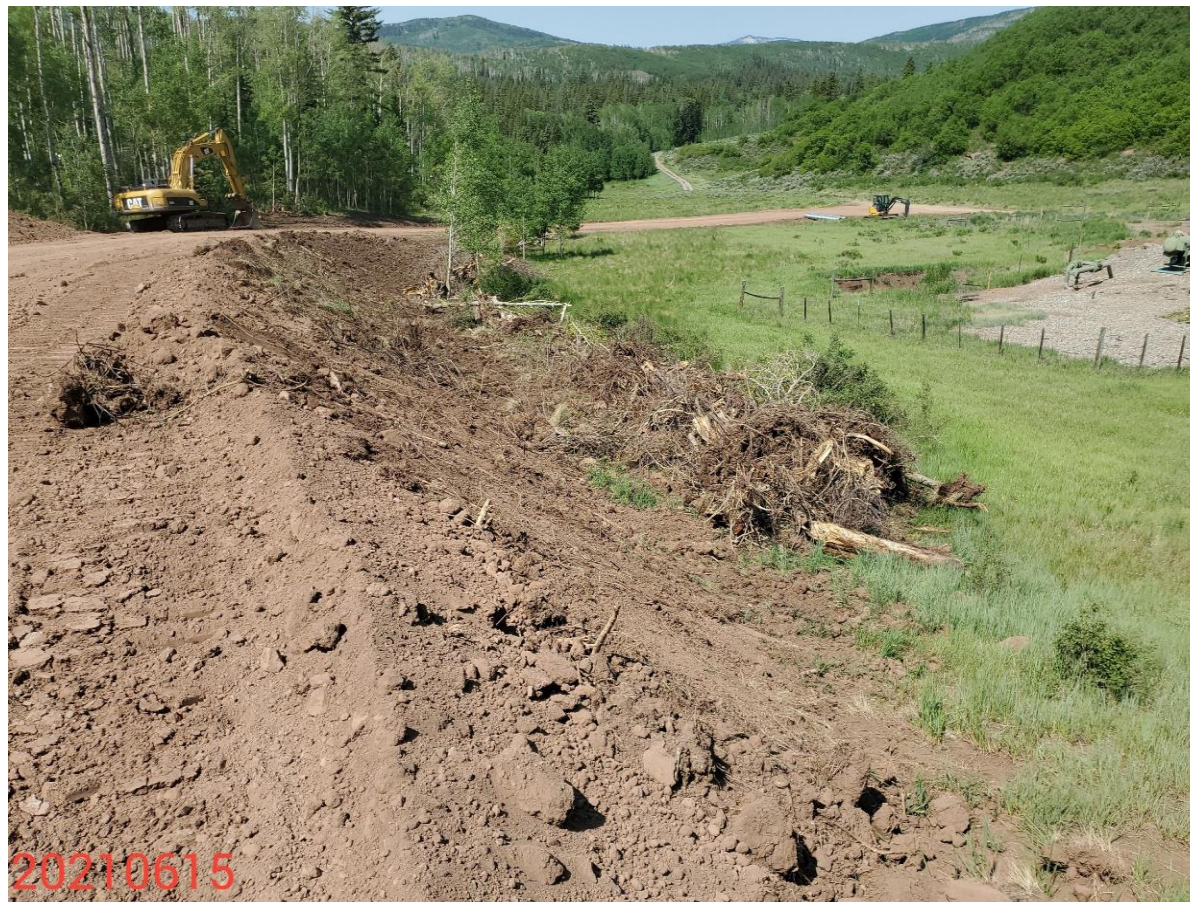
Photo 26: Photo shows Stormwater erosion control BMPs to prevent off site sediment transport, and to stabilize the slopes along the access road remain missing or insufficient.
