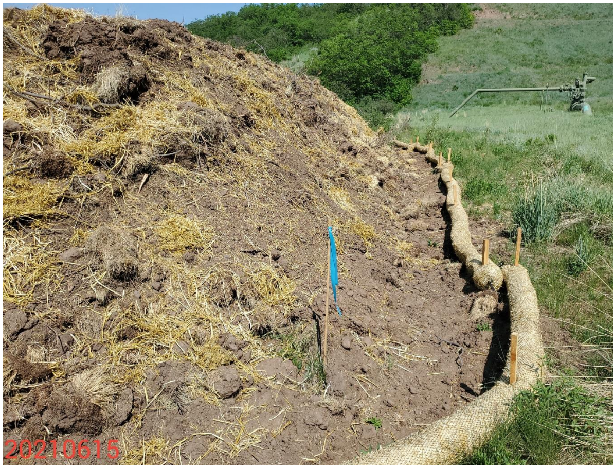
Photo 6: Photo taken from the topsoil stockpile on the north end of the Location. Photo shows Operator has applied a straw mulch onto the soil stockpile, and installed erosion logs at the base of the stockpile. Straw has not been crimped, or used in conjunction with any other stabilization BMP, and is insufficient alone to stabilize and protect the topsoil stockpile.
