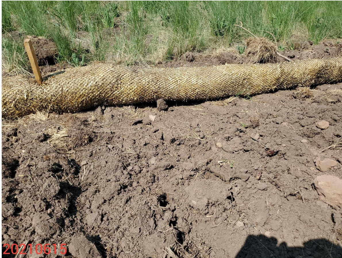
Photo 28: Continued from photo 22. Erosion logs have not been installed in accordance with good engineering practices; logs have only been placed onto the top of the soil and staked; erosion logs have not been properly trenched and backfilled.
