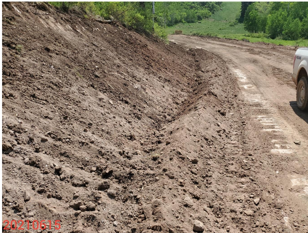
Photo 24: Photo shows control measures to protect/stabilize the cut slopes along the access road are missing or insufficient.
