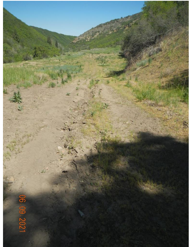
Photo#4: Erosion on road at Southeast end of site.
