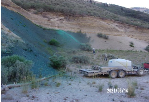
Applying Additional Water, Nutrients, and Soil Amenities on CC 629-23-42 Cut Slope
