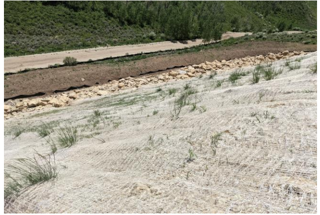
Desirable Vegetation Growing through Jute Netting on CC 604-12-13 Annex Pad
