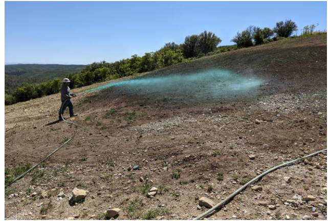
Applying Liquid Soil Amenities on CC 604-12-13 Annex
