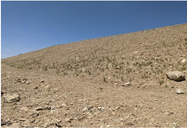
Desirable Vegetation Growing on Upper Section of Fill Slope on CC 604-12-13 Annex Pad
