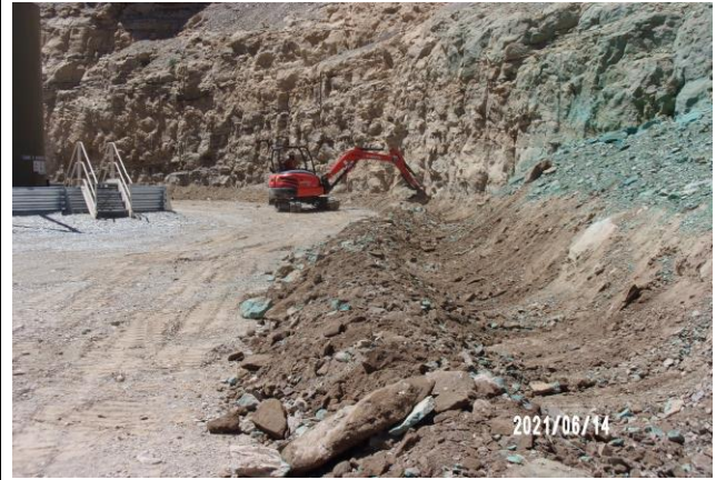
Installing Containment Berm Below CC 604-12-13 Annex Cut Slope
