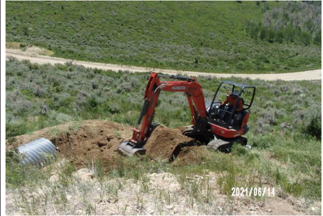
Installing Outlet Protection on Culvert on CC 604-12-13 Annex Access Road
