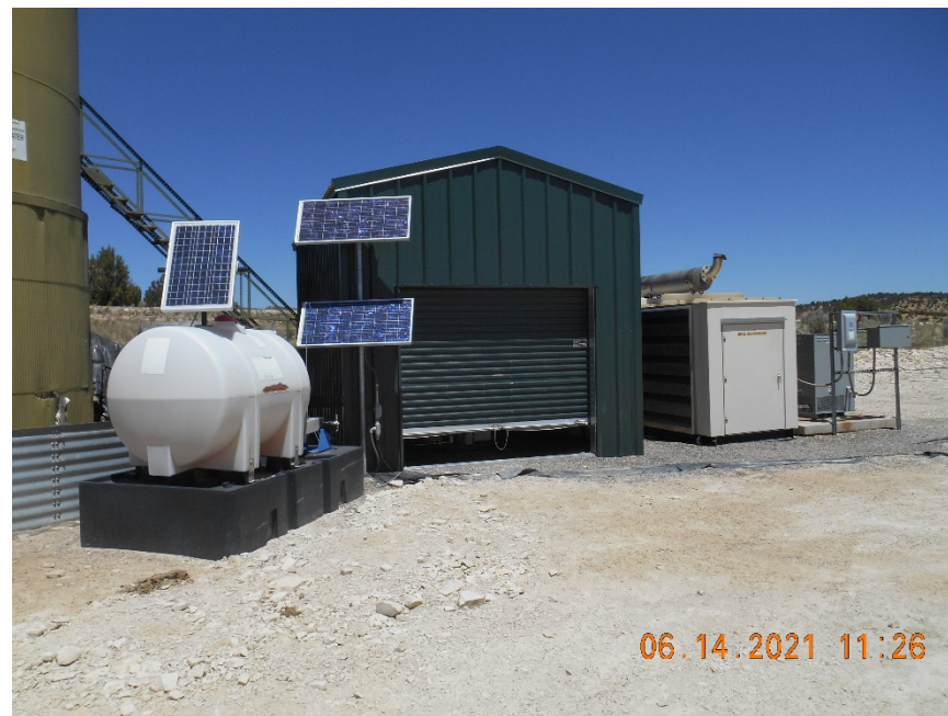
Pump Housing. Chemical injector with secondary containment.
