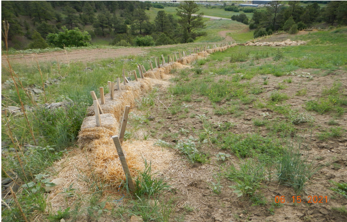
Photo 8. There are straw bales around the perimeter that have degraded. The bales should be removed or replaced if needed.
