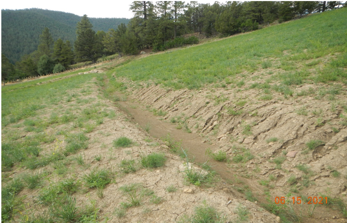
Photo 10. Facing southwest along the reclaimed location. There is a diversion berm along this area which could use some maintenance and hand seeding.
