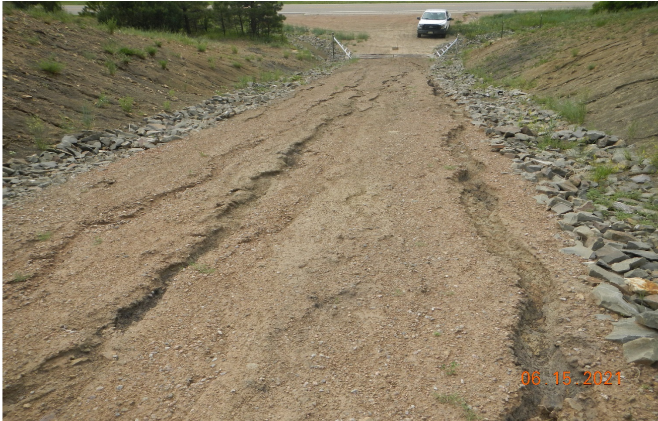
Photo 3. Facing back along the access road. Stormwater should be diverted off the road to prevent erosion.
