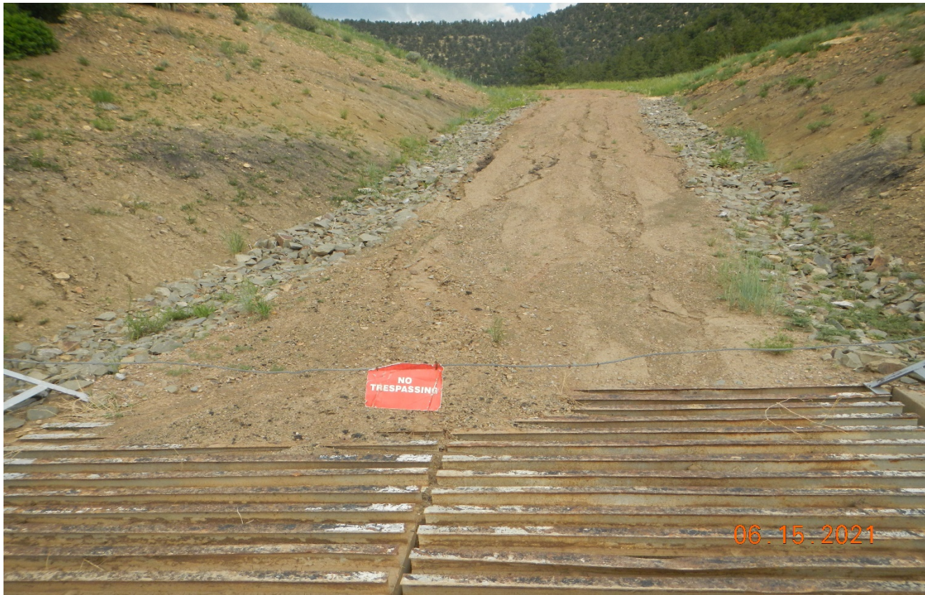
Photo 1. Facing north toward the access road. There is some sediment beginning to fill into the cattle guard.
