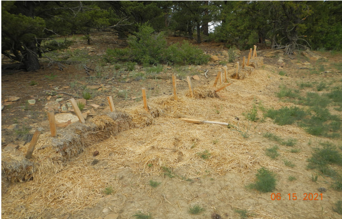
Photo 13. There are straw bales around the perimeter that have degraded. The bales should be removed or replaced if needed.
