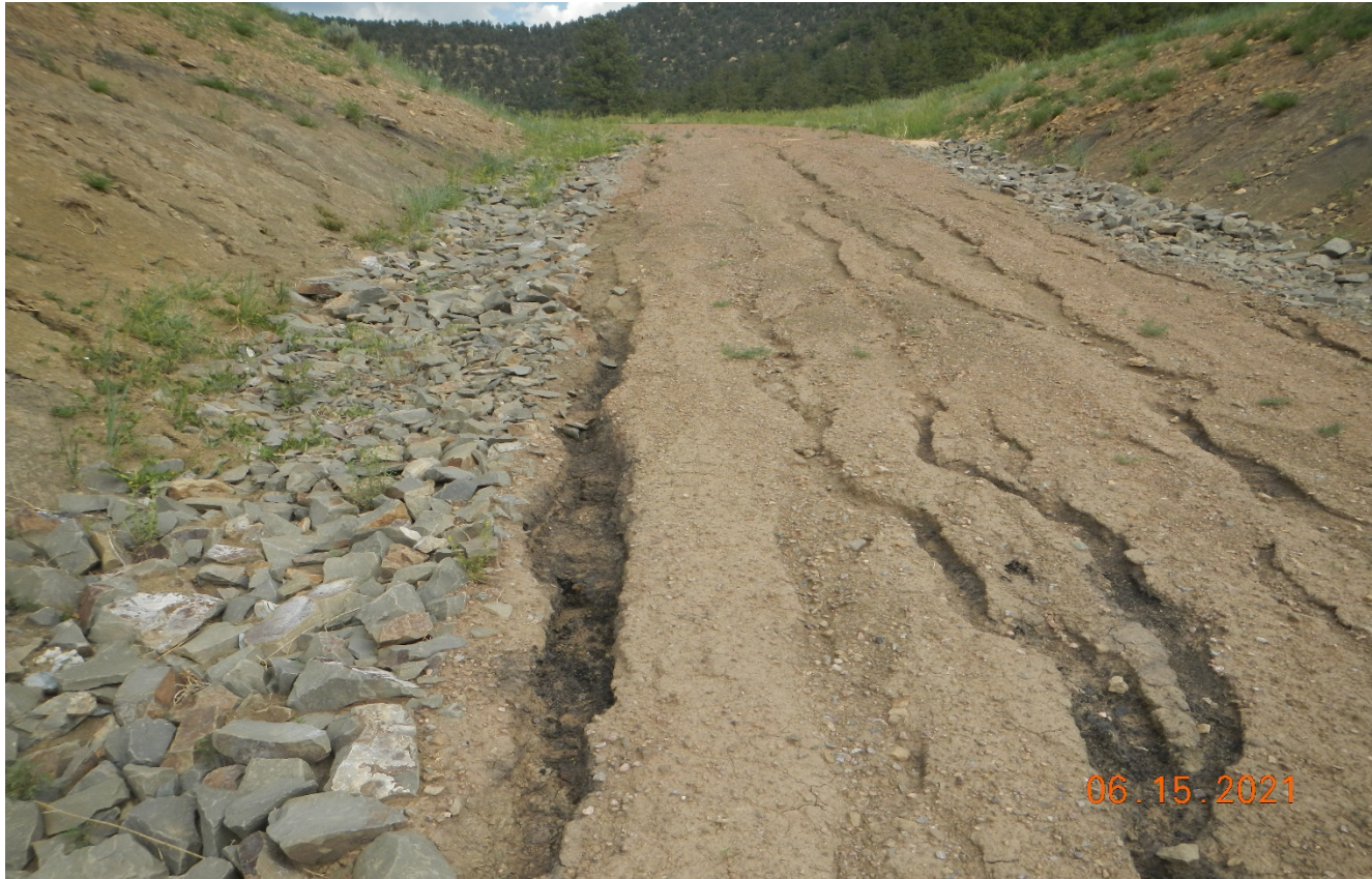
Photo 2. Stormwater is causing erosion at the beginning steep grade of the road. Storm water should be diverted off the road to prevent erosion (berm, water bar).
