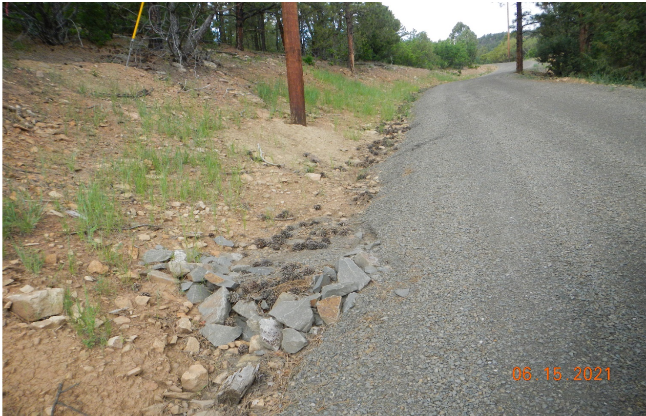
Photo 4. Sediment has accumulated on some of the check dams which need maintenance.
