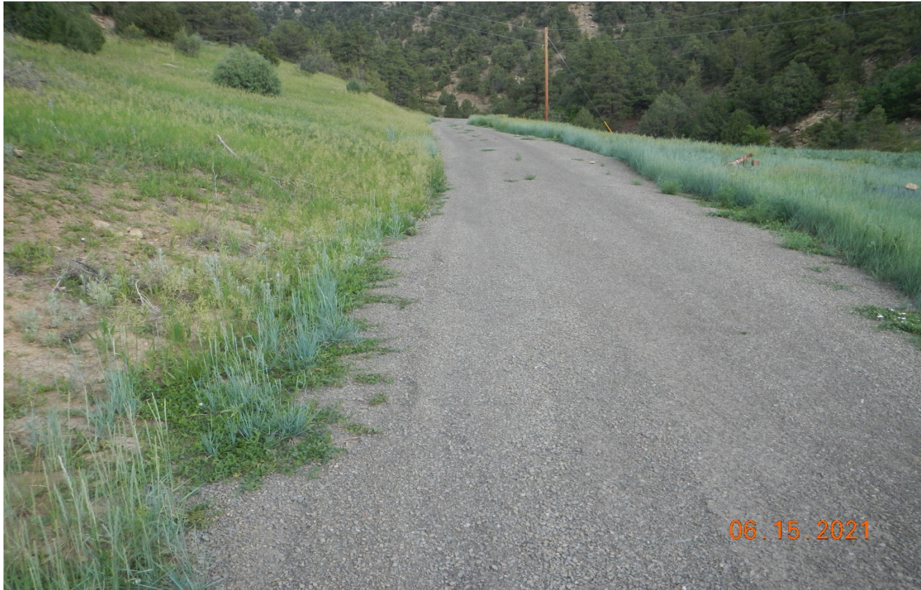
Photo 1. Facing north toward the access road. Gravel has been spread along the road for stabilization.
