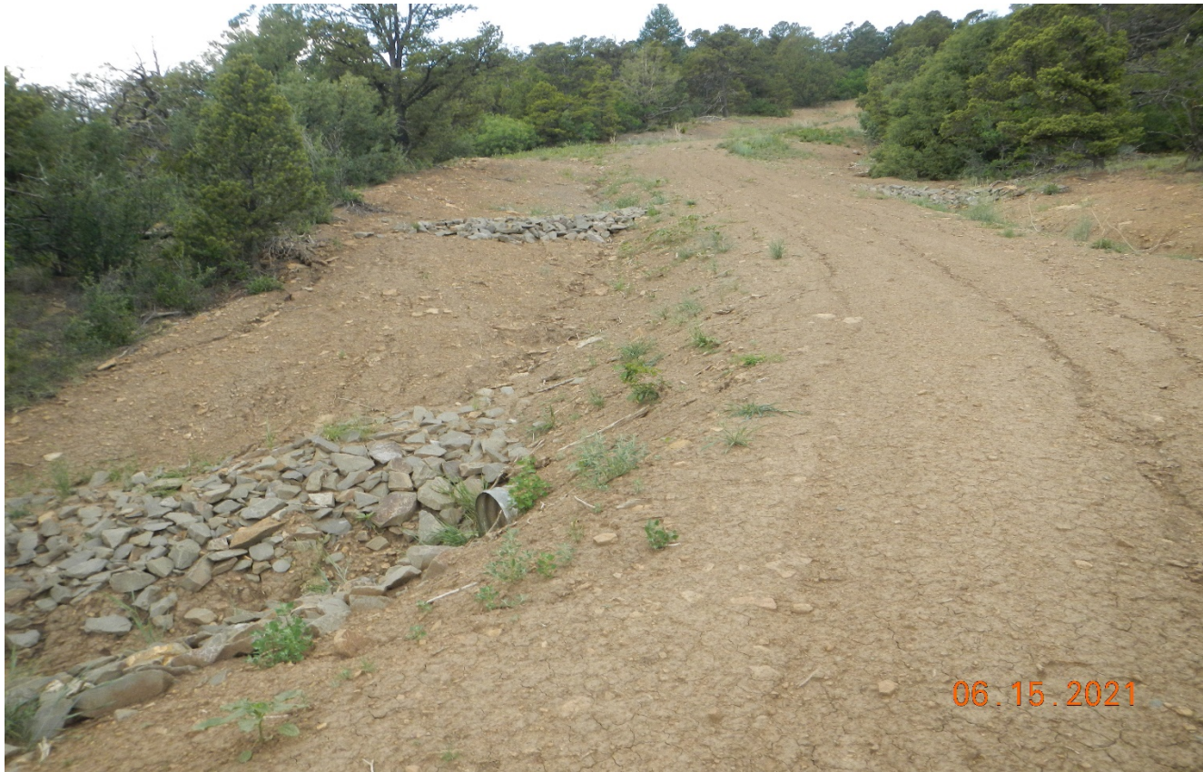
Photo 7. Facing northwest along the road. Culverts are installed along the road.
