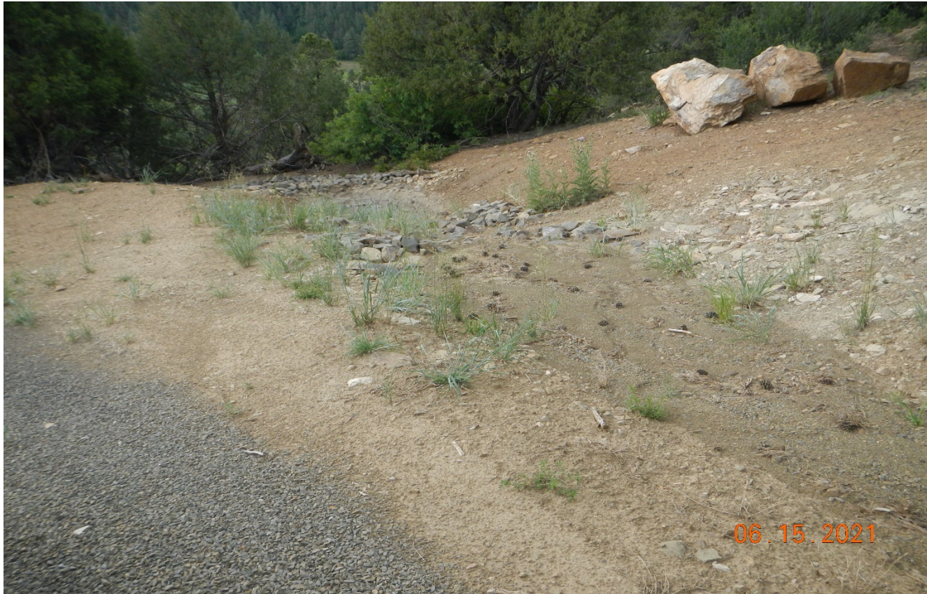
Photo 2. There is sediment accumulation along this rip/rap outlet which needs maintenance.
