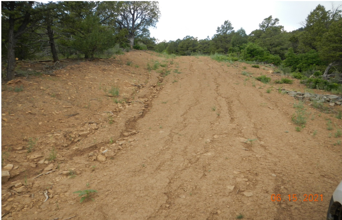
Photo 6. Facing northwest. There is erosion beginning to occur which needs maintenance.
