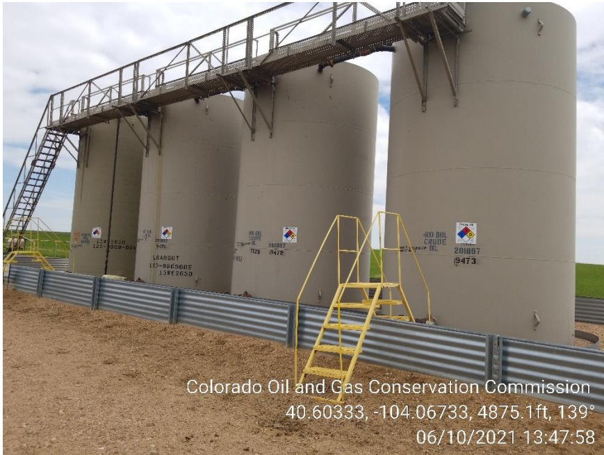
Photo 11 – Tank Battery
