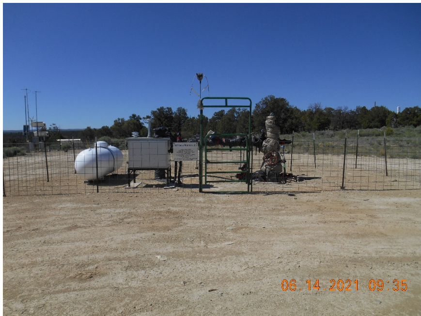
Injection wellhead & line heater
