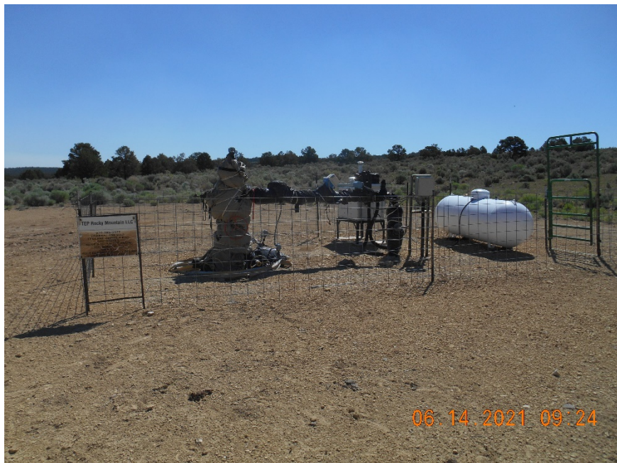
Injection wellhead & line heater
