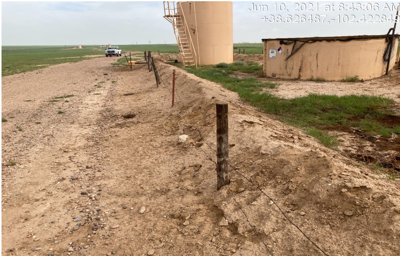
Photo 4. The fence is not maintained around the tank battery to prevent livestock entry. Cattle tracks are shown along the berm.
