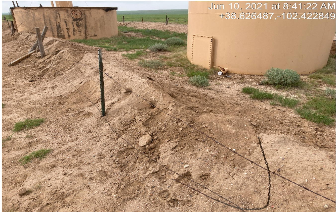
Photo 2. The fence is not maintained around the tank battery to prevent livestock entry. Cattle tracks are shown along the berm.
