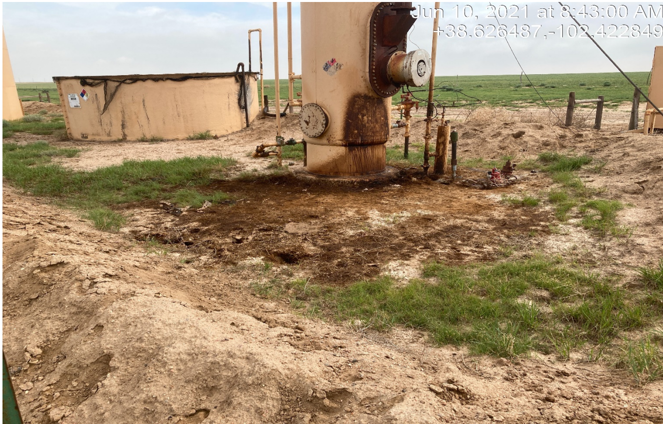
Photo 3. There is oil stained soil around the tank. The stained soil needs to be cleaned up.
