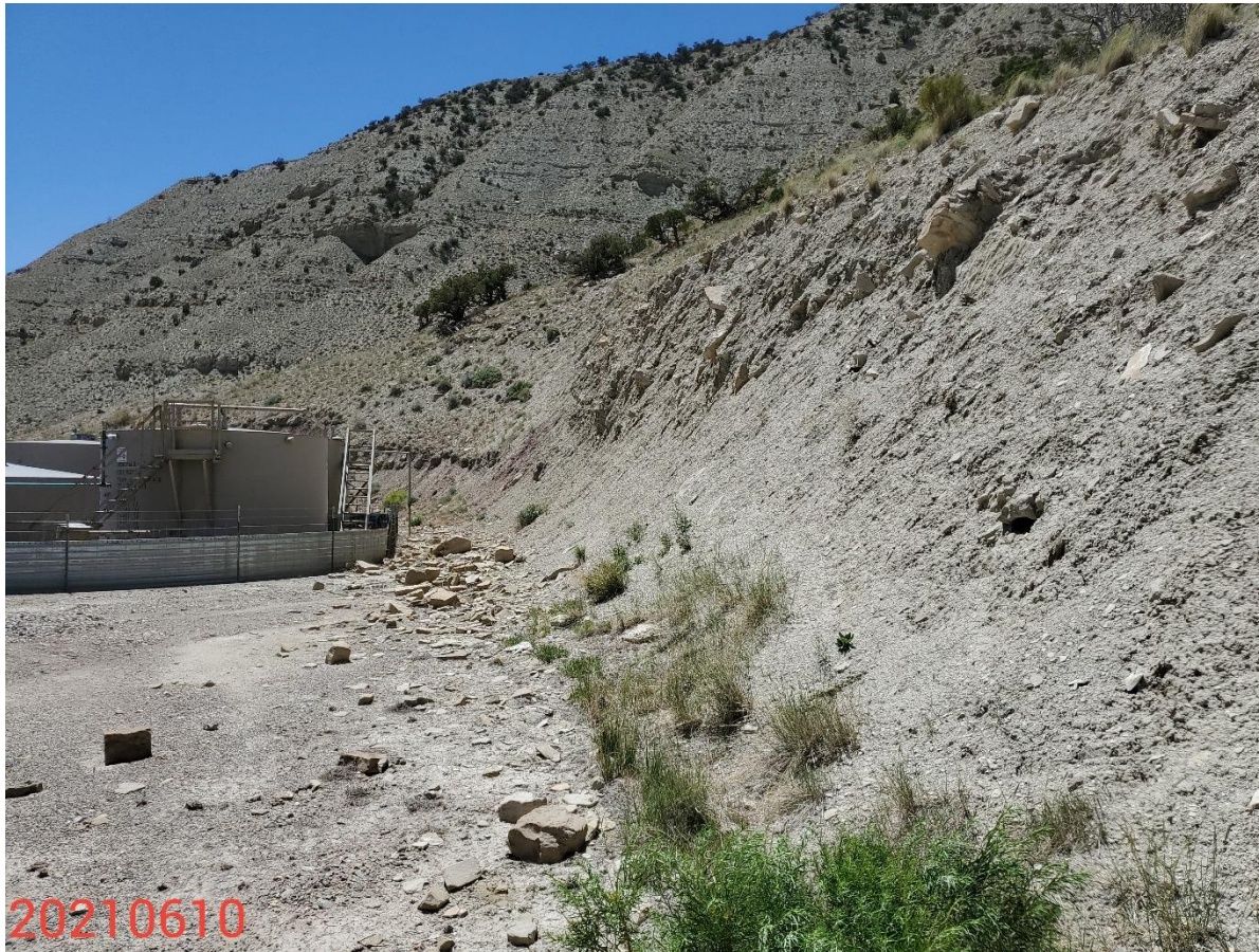
Photo 5: Photo taken from the cut slopes on the north end of the Location. Photo shows control measures to protect and stabilize the cut slopes of the Location remain missing or insufficient; corrective action not addressed
