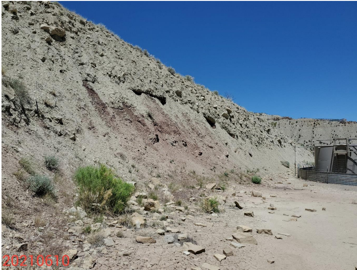
Photo 3: Photo taken from the cut slopes on the north end of the Location. Photo shows control measures to protect and stabilize the cut slopes of the Location remain missing or insufficient; corrective action not addressed
