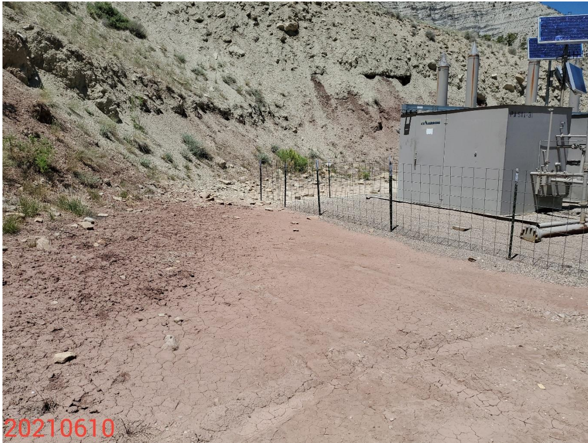
Photo 2: Photo taken from the cut slopes on the north end of the Location. Photo shows control measures to protect and stabilize the cut slopes of the Location remain missing or insufficient; corrective action not addressed
