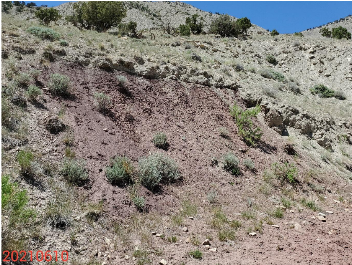
Photo 1: Photo taken from the cut slopes on the north end of the Location. Photo shows control measures to protect and stabilize the cut slopes of the Location remain missing or insufficient; corrective action not addressed
