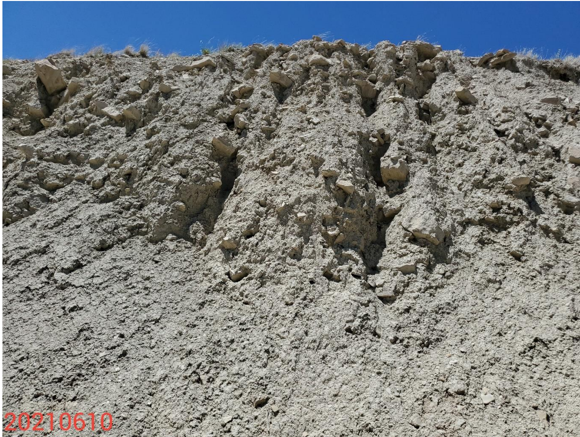
Photo 4: Photo taken from the cut slopes on the north end of the Location. Photo shows control measures to protect and stabilize the cut slopes of the Location remain missing or insufficient; corrective action not addressed
