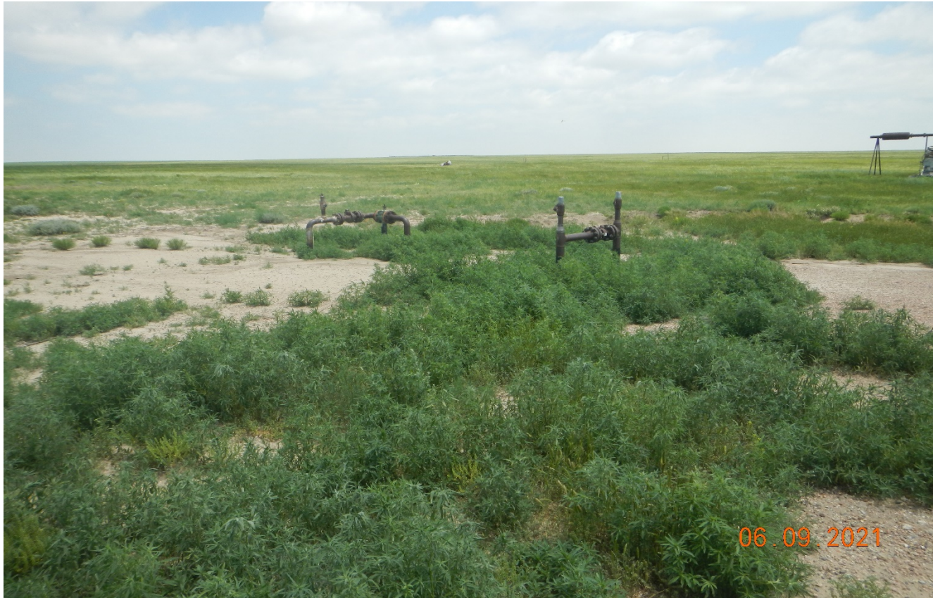
Photo 2. Abandoned pipe risers have not been removed.
