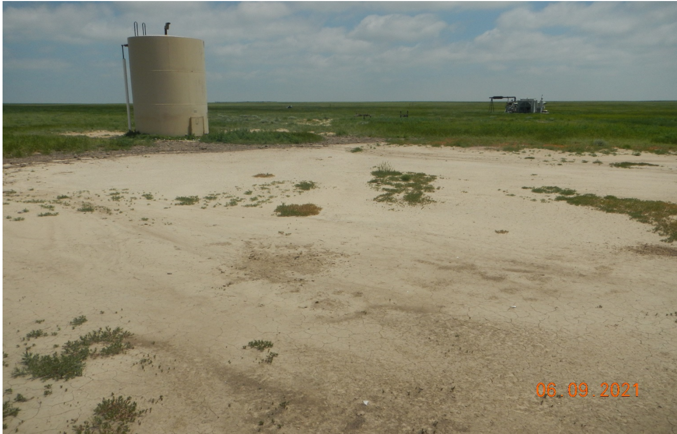
Photo 1. Facing northeast at the location. Tank has not been removed and soils have no vegetation growth indicating a potential spill area.
