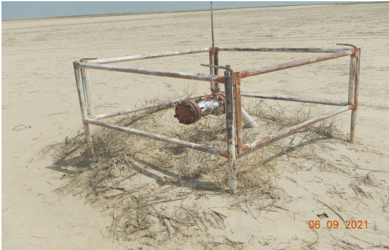
Photo 2. View of pipeline riser at the location. No sign identifying the riser is present.
