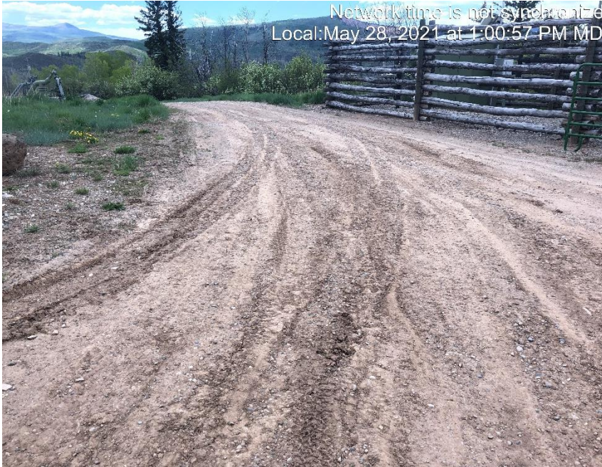
Photo #3979 No form of tracking BMP located at the entrance to location.
