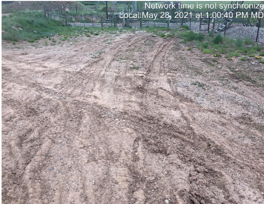
Photo #3977 Location lacks stabilization.
