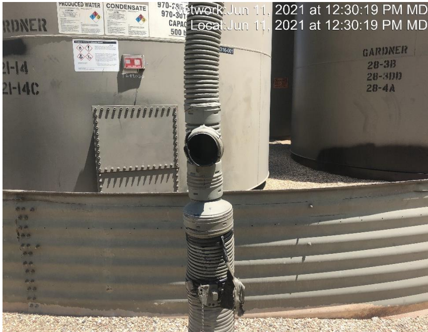
Photo #4073 Multiple flow line heating insulation open ended and not capped.
