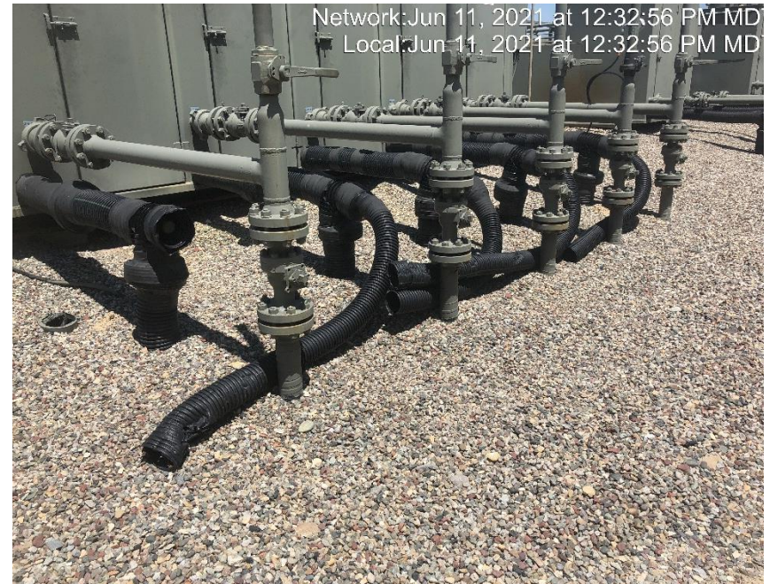
Photo #4074 Multiple flow line heating insulation open ended and not capped.
