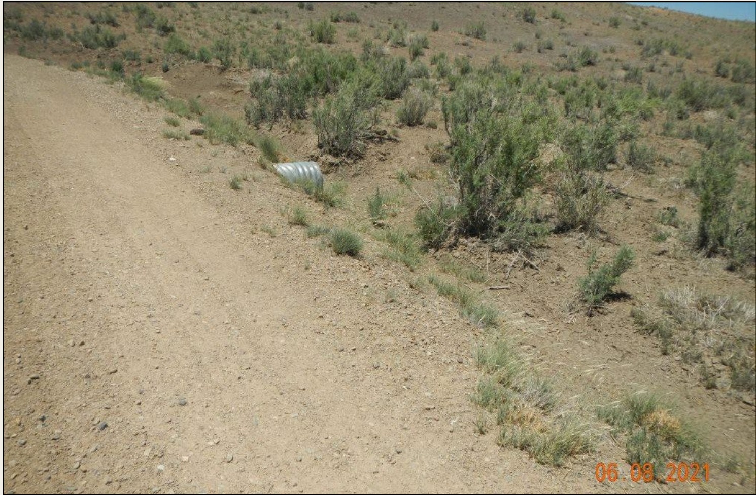
Photos 3. View of culvert inlet along the access road.
