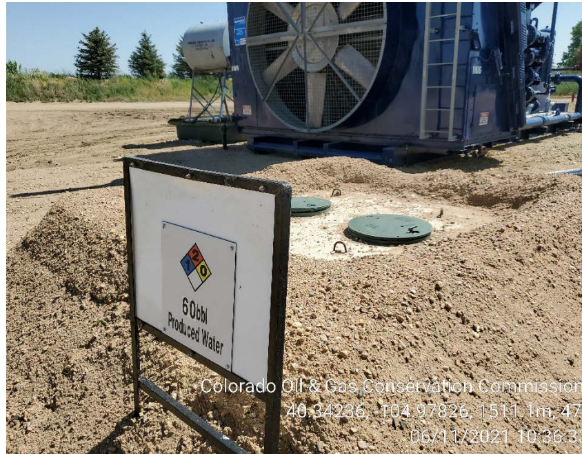
Produced water tank berm
