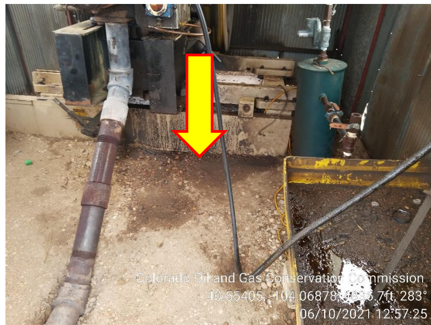
Photo 6 – Stained Soil at Gas Engine
