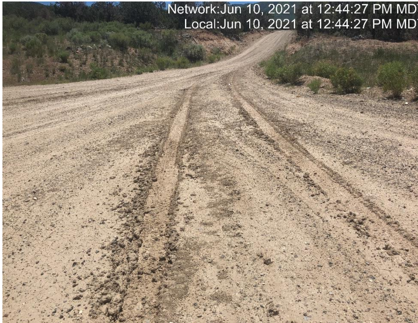
Photo #4054 No form of tracking BMP located at entrance to location.
