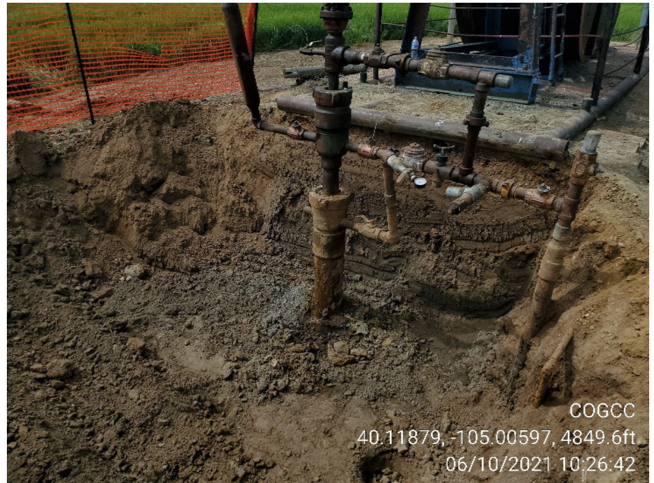
Photo 2 Excavation around wellhead and casing
