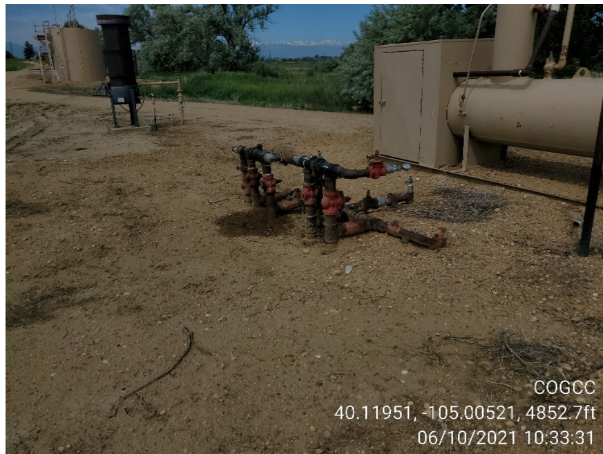
Photo 5 Leak at piping header at tank battery
