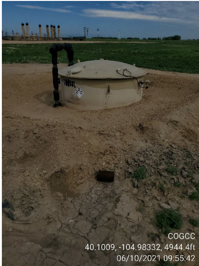
Photo 3 Produced water vessel and containment berm
