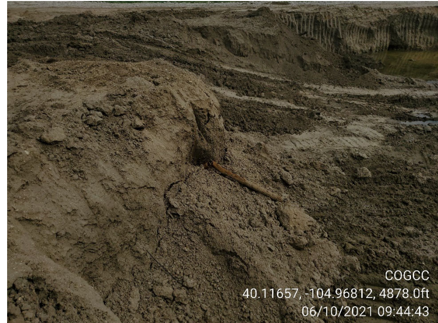
Photo 6 Flowline or dumpline piping in western wall of eastern excavation
